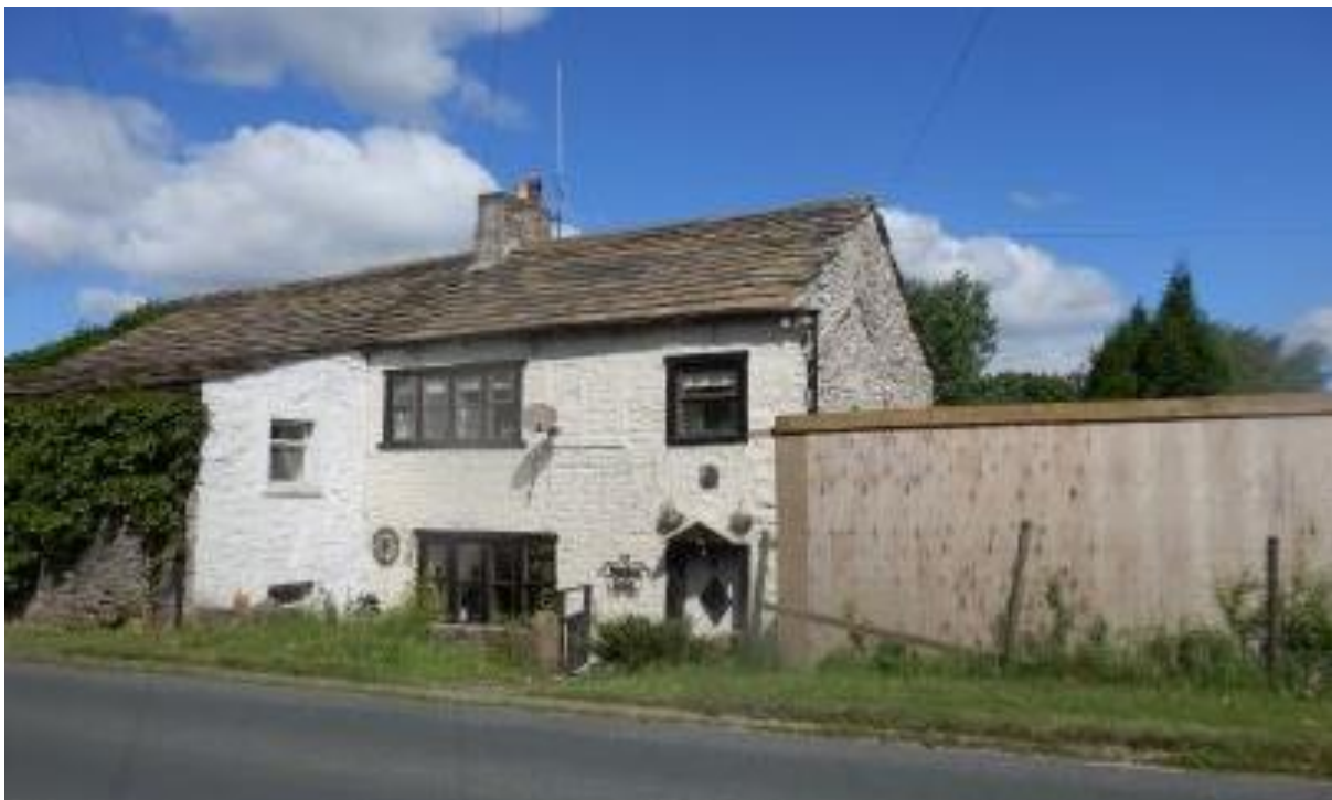
Image 1 Nuttercote Cottage as at June 2018. Nuttercote Farm was to the right of the property before its demolition.
