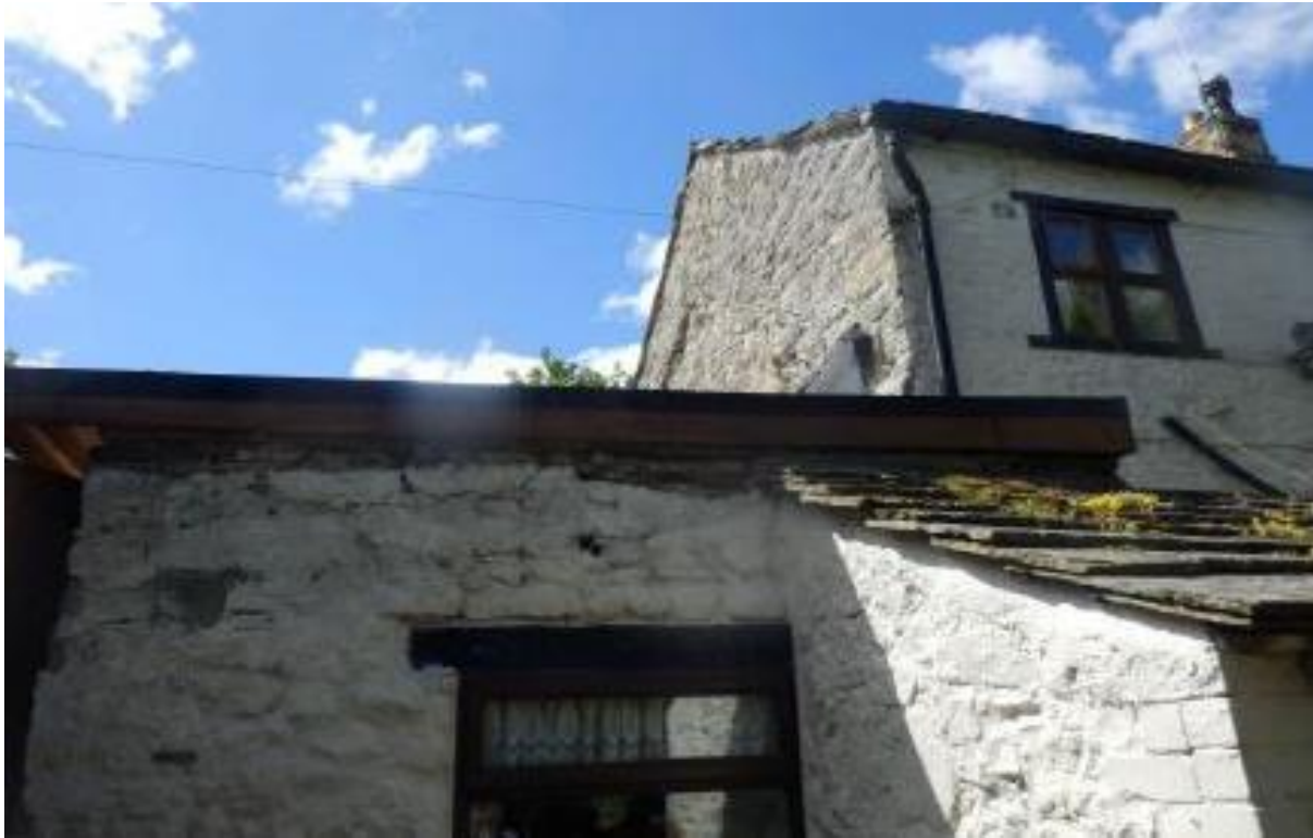
Image 4 Lean to and rear of the Dining Room with temporary roof over above.
