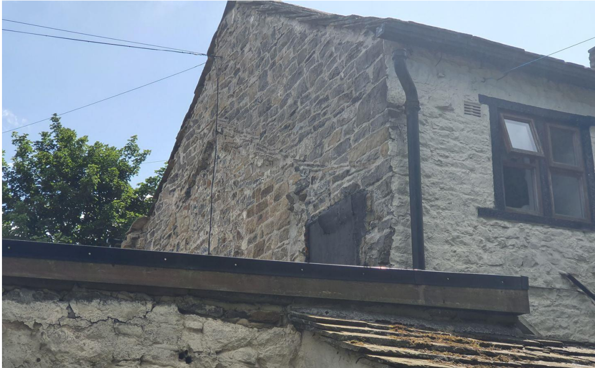
Closer view looking towards North Elevation
