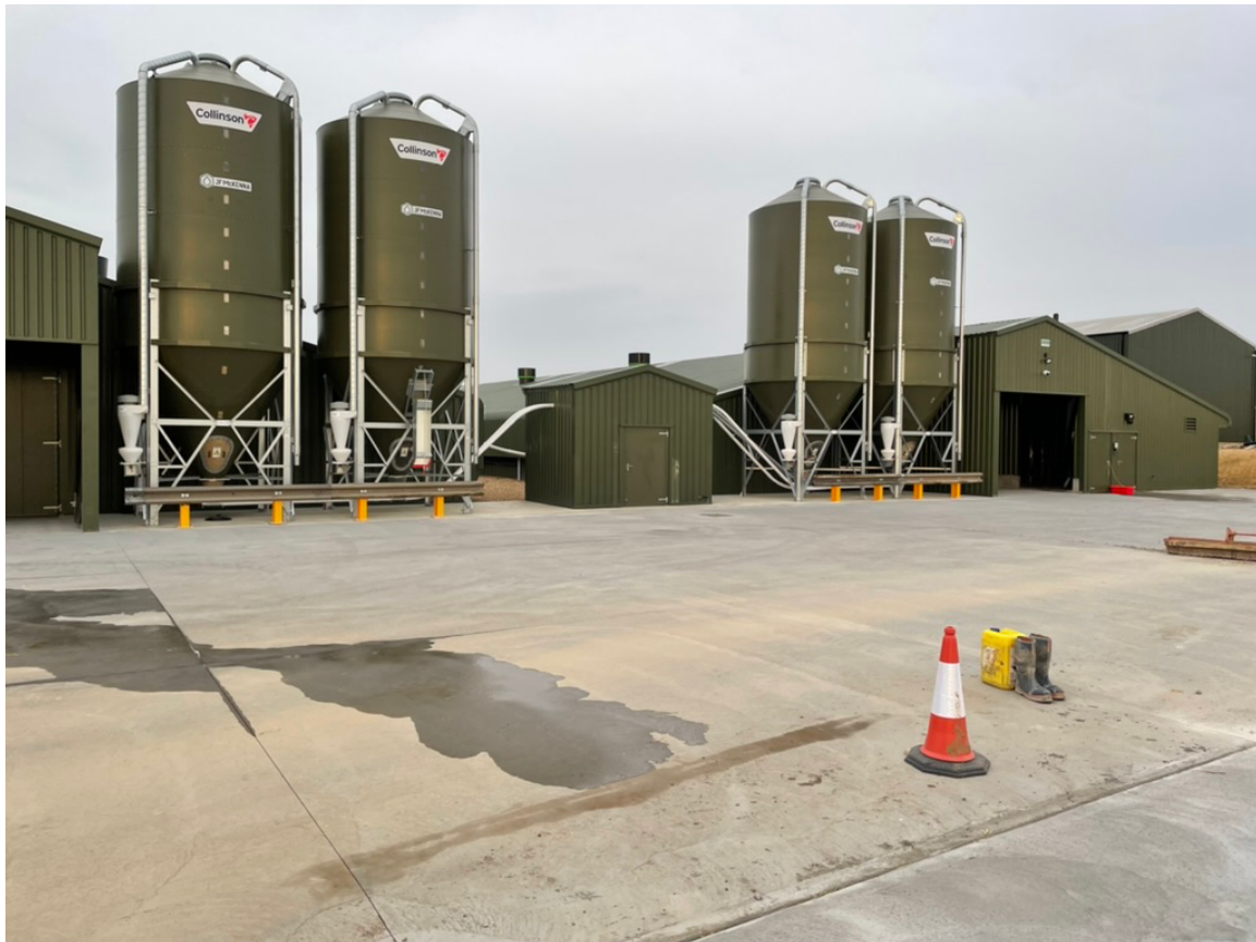
Photo 1. This photograph shows the existing buildings on the site.
