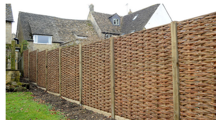
Fence Type 3 (F3): Front Drive, Bin Store & Oil Tank 1.8m high 'Heritage' framed willow fence, to match existing & to replace degraded willow fence; to screen bins & oil tank. Supplier: Winterbourne Willows
