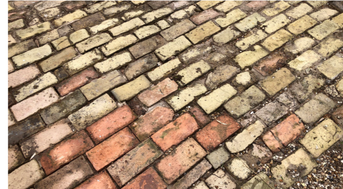
Rear Garden Courtyard: Existing bricks reclaimed, cleaned & reinstated (Loading Class as required)
