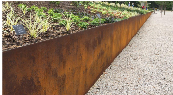
Edge Type 1 (E1): Vehicular Access Track Embankment Option 01: Untreated steel edge, 6mm; up-stand varies up to 500mm. Supplier: Contractor to propose local supplier
