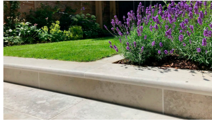
Rear Garden Terrace Steps: Jura Grey Smooth Limestone Bullnose Step, 1200/900x600x40mm (Loading Class as required). Supplier: London Stone
