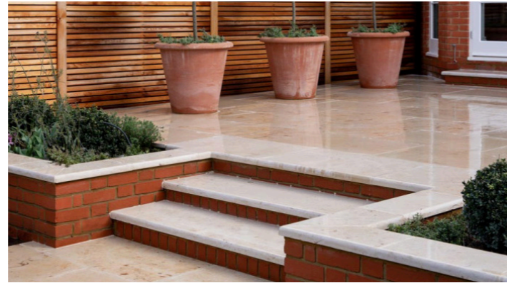
Wall Type 2 (W2): Rear Garden Terrace Retaining Wall Option 01: 450mm high, Red brick retaining wall, with Jura Grey Smooth Limestone coping Supplier: London Stone (coping); brick: contractor proposed
