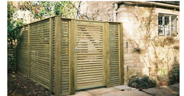
Gate Type 4 (G4): Rear Garden Log Store Enclosure 1.78m high, Venetian Gate, 1000mm width; FSC timber, to match Fence Type 4. Supplier: Jacksons Fencing
