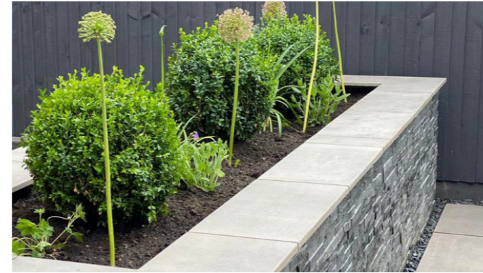
Wall Type 2 (W2): Rear Garden Terrace Retaining Wall Option 02: 450mm high, limestone clad retaining wall, with Jura Grey Smooth Limestone coping. Supplier: London Stone
