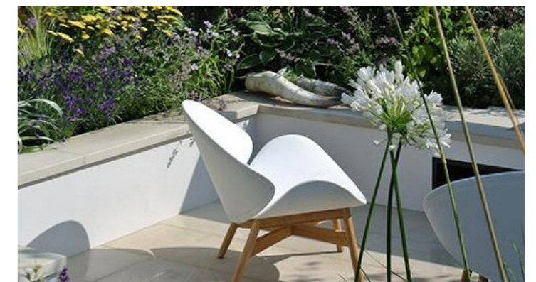
Wall Type 2 (W2): Rear Garden Terrace Retaining Wall Option 03: 450mm high, pale grey rendered retaining wall, with Jura Grey Smooth Limestone coping. Supplier: London Stone
