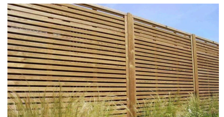
Fence Type 4 (F4): Rear Garden, NW & SE Boundaries, Log Store Enclosure 1.83m high FSC timber 'Venetian', horizontal slatted fence. Supplier: Jacksons Fencing
