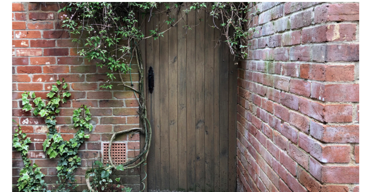
Wall Type 4 (W4): Rear Garden Courtyard Extension to existing brick boundary wall; brick, piers, coping & height to match existing (to Architect's specification)
