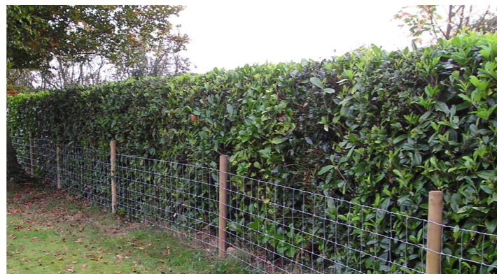
Fence Type 2 (F2): Rear Garden, SE Boundary 1.2m high timber post & galvanised wire dog-proof fence (concealed within proposed boundary hedge). Supplier: Contractor to propose local supplier
