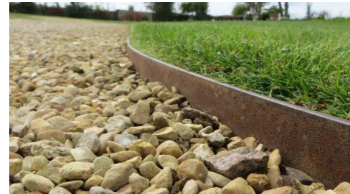
Edge Type 2 (E2): Drive Gravel / Soft Landscape Interface: Untreated steel edge, 6mm; 100mm up-stand. Supplier: Contractor to propose local supplier
