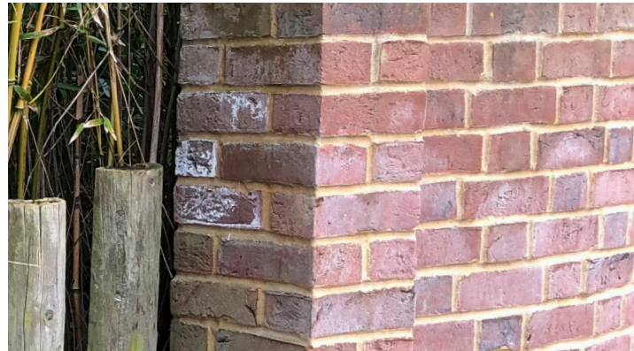
Wall Type 1 (W1): Front Garden Drive Boundary & Entrance Extension to existing brick boundary wall; brick, piers, coping & height to match existing (to Architect's specification)
