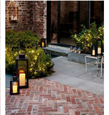
Terraces & Paths: Muted red "Dutch" clay paver, 200x48x58mm or 210x100x50mm, half-lap stretcher & herringbone bonds, with single/triple row running bond margins (Loading Class as required). Supplier: London Stone
