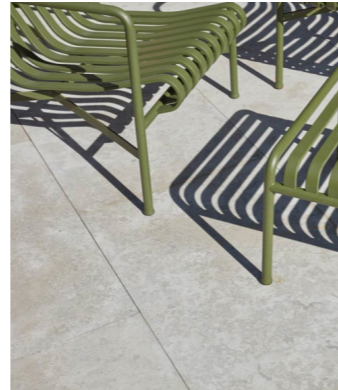
Terraces & Paths: Jura Grey Smooth Limestone paving, 900x600x22mm, 600x600x22mm & 600x400x22mm (Loading Class as required). Supplier: London Stone
