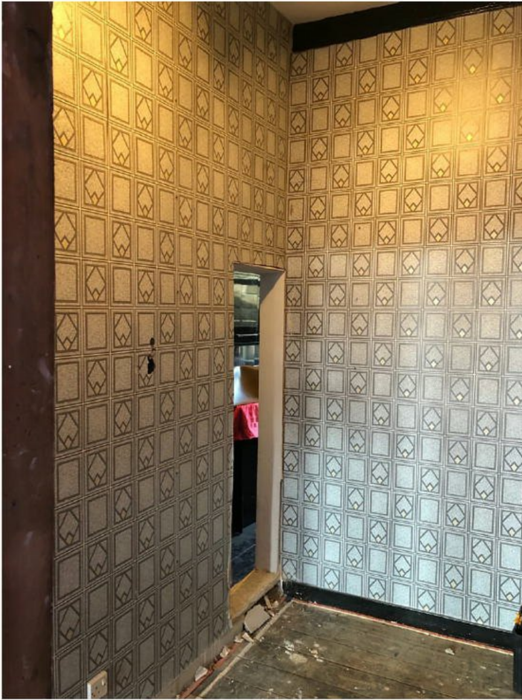
Cupboard space showing current access to kitchen
