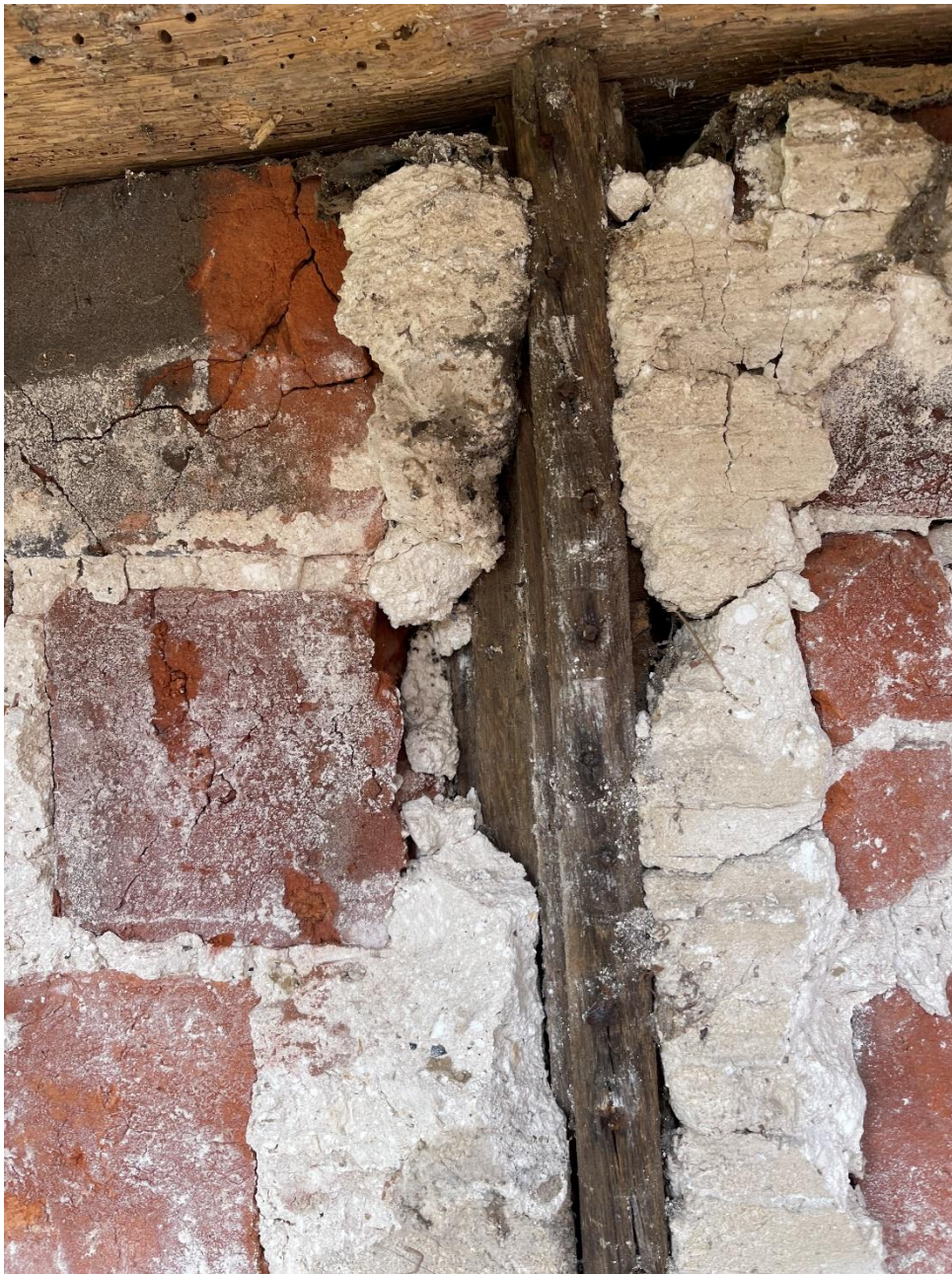
Close up picture of the mullion
