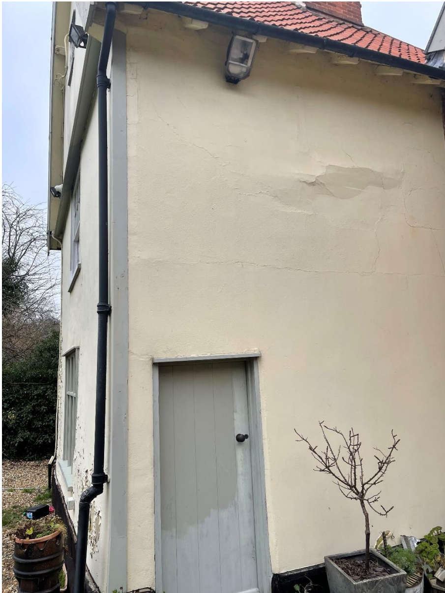
Picture of the wall before render was removed.
