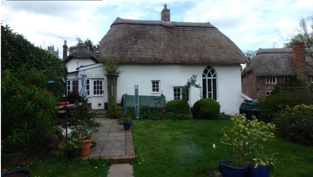
View from the south
