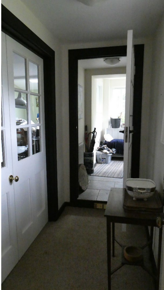
The partition 2 on the left is to be removed.
