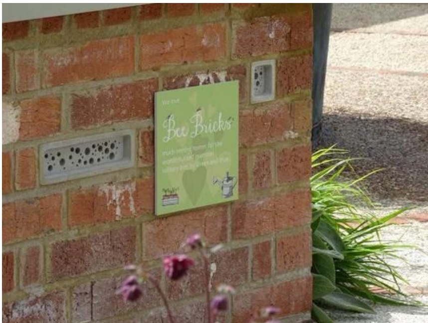
Bee brick & bee block incorporated into an external brick wall
