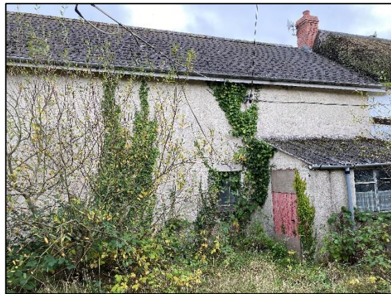
Plate 12: Rear of 3 Leigh Cross (facing south-west)
