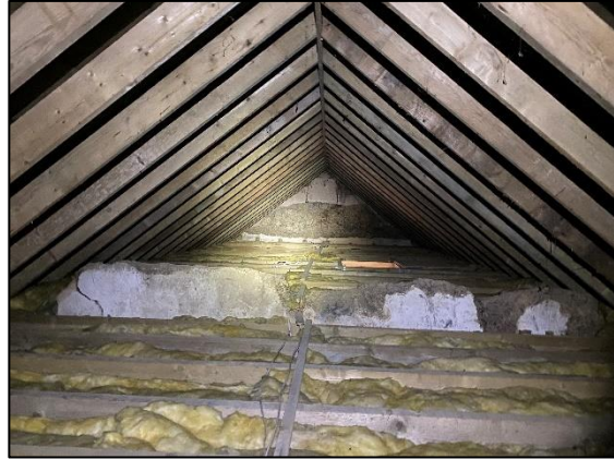
Plate 6: View of loft void of 3 Leigh Cross
