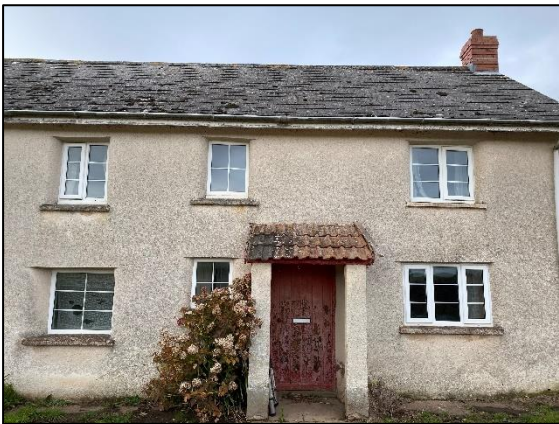
Plate 11: Front of 3 Leigh Cross (facing north)
