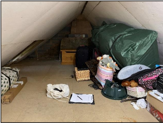
Plate 1: View of roof void (facing west)
