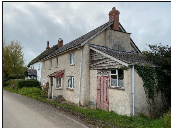
Plate 14: View of 3 Leigh Cross (facing north-west)
