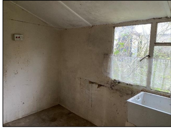
Plate 10: Ground floor lean-to (facing north-west)
