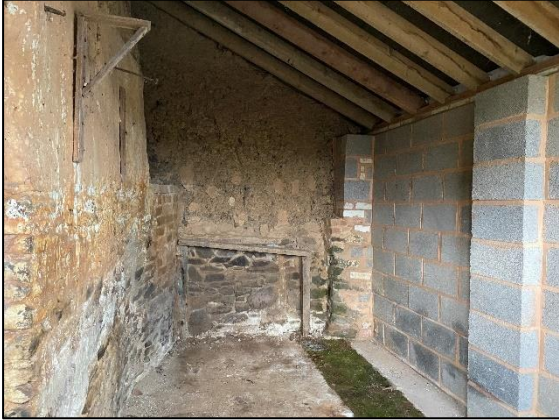
Plate 15: View inside store (facing north)
