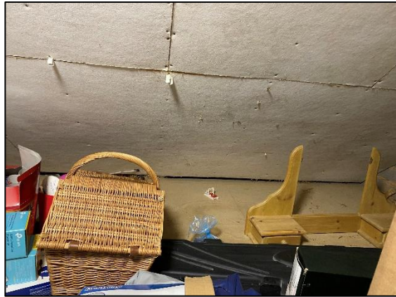
Plate 2: Underside of roof
