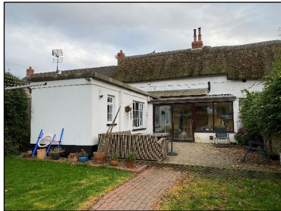
Plate 4: Rear of 2 Leigh Cross (facing south-east)
