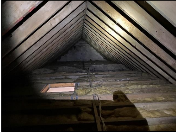
Plate 5: View of loft void of 3 Leigh Cross
