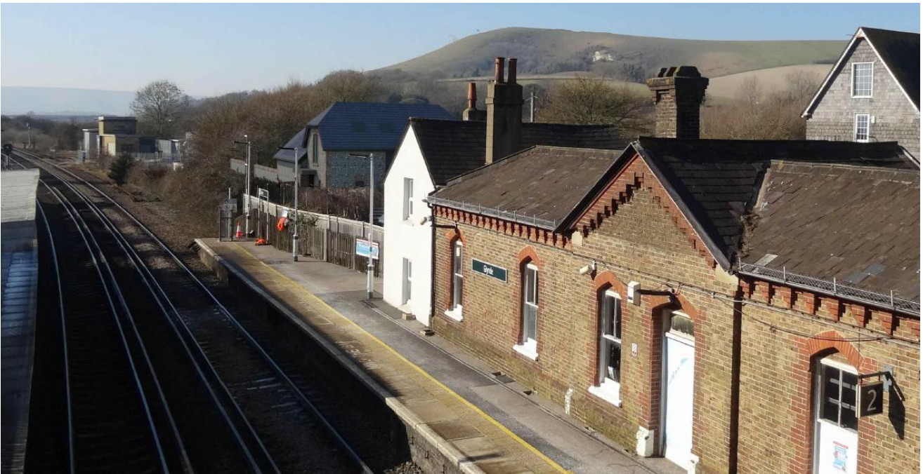
3D render of south elevation – taken from the bridge that crosses the railway line:
