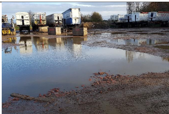
Photograph 5: Hardstanding and mud areas in centre of site.
