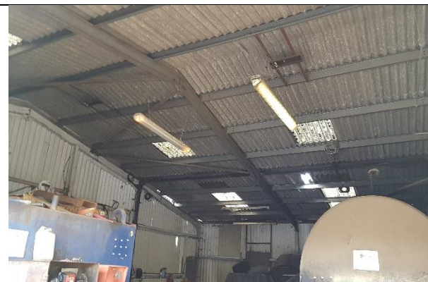
Photograph 4: Unlined roofs of metal framed units.
