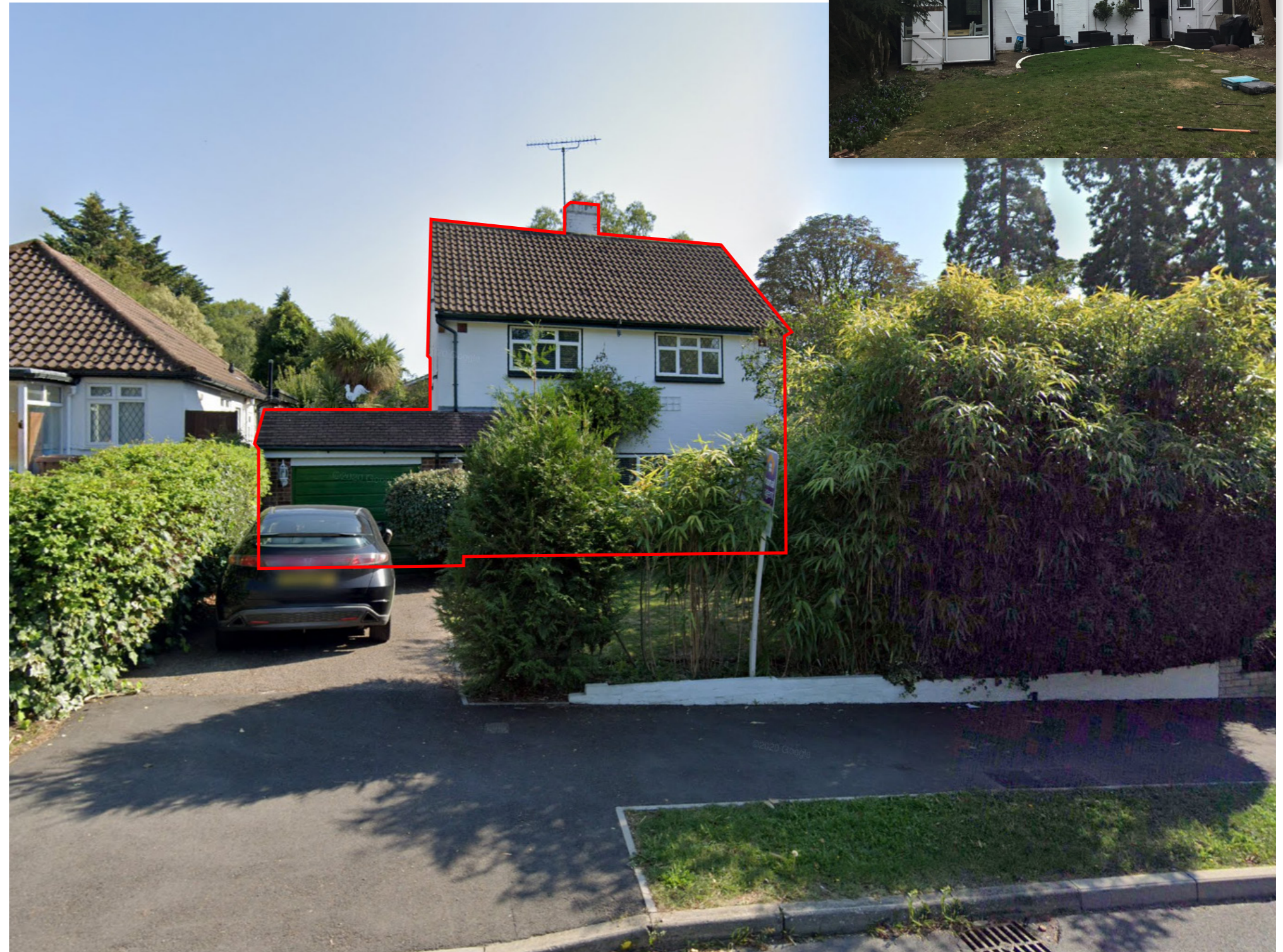
View of the existing property from the street (red outline)
