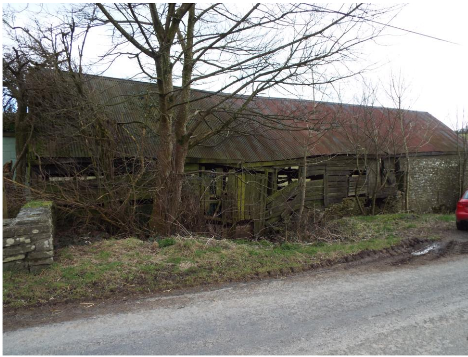
Figure 2 : NW elevation to roadside.
