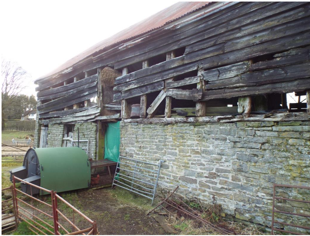
Figure 6 : SE flank walling.
