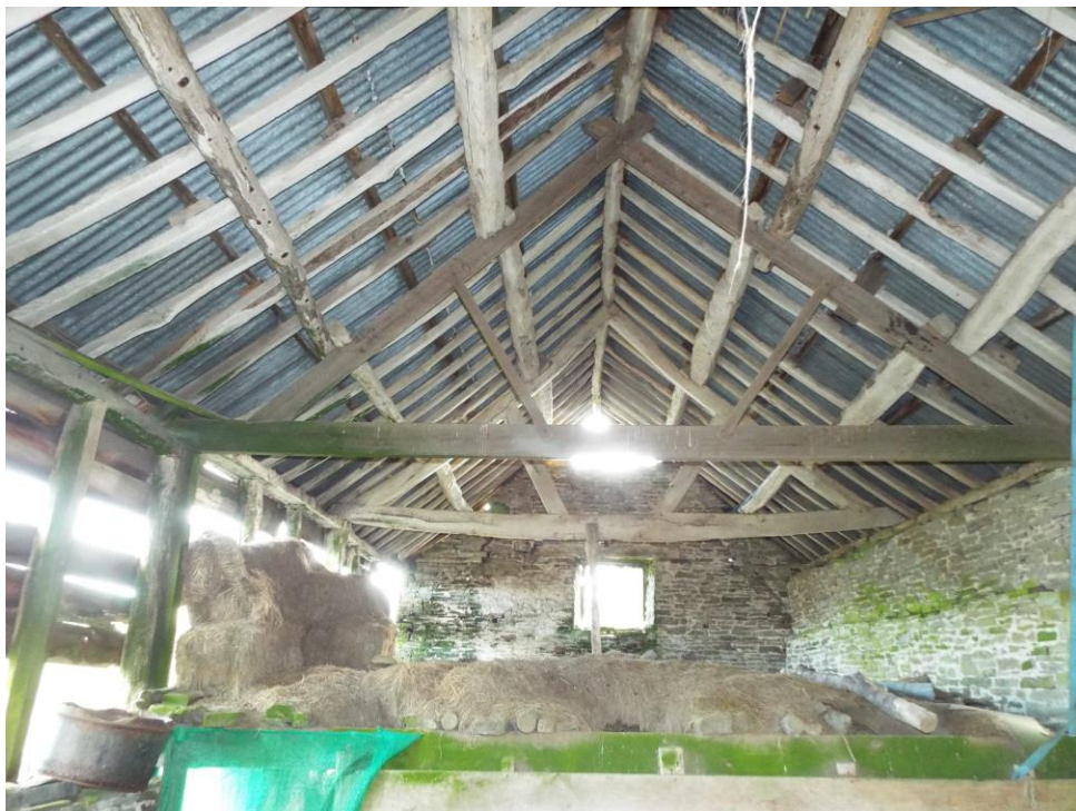
Figure 12: Mezzanine bays view S.
