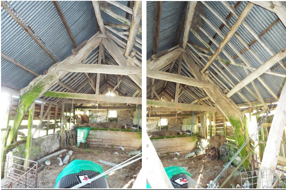
Figure 11: Cruck bay view south.
