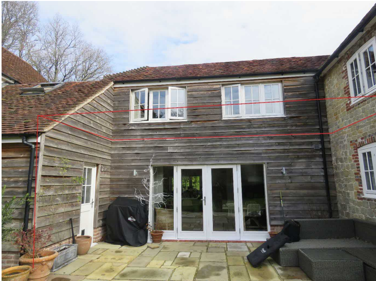
Figure 3. Showing proposed location of proposed orangery / garden room. Red lines are indicative of proposed extent, ceiling height being approximately 3-4 boards below the upper storey windows.
