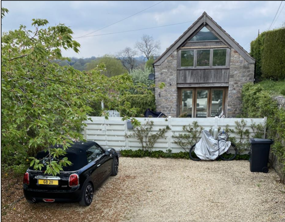
The Barn (exterior end elevation)
