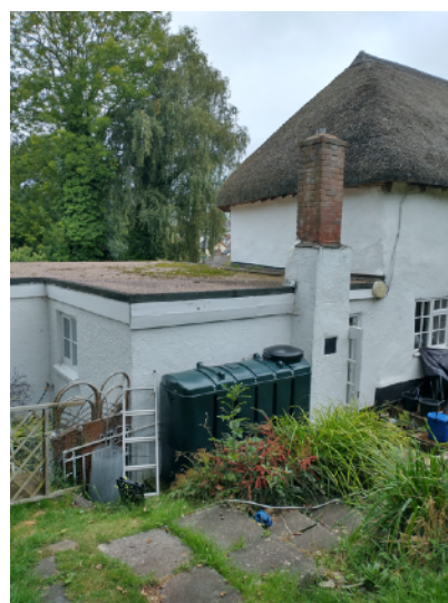
Existing chimney stack
