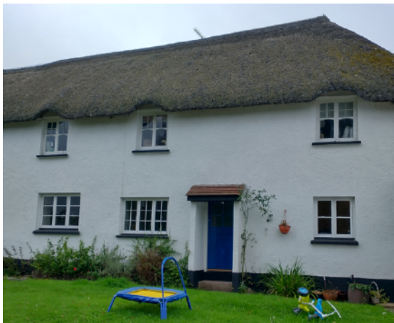
Front of cottage with curved window fenestration
