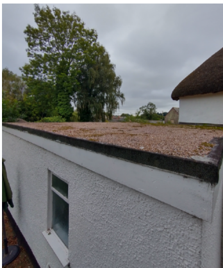
Existing flat roof
