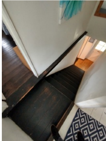
Mechanical cut staircase
