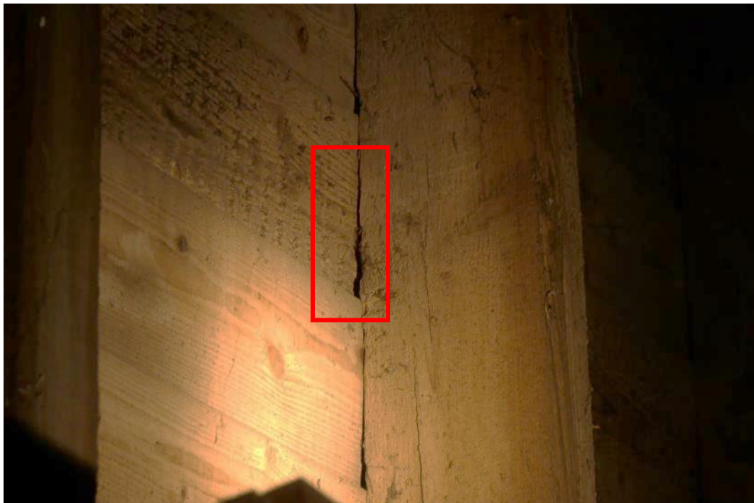
Photo 5 , common pipistrelle roost location on the south aspect of the main barn highlighted in red. 4 th May 2022.
