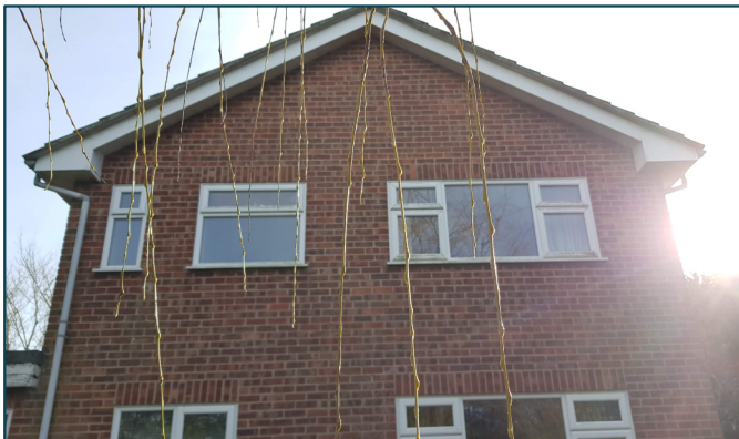
Rear (north west)
