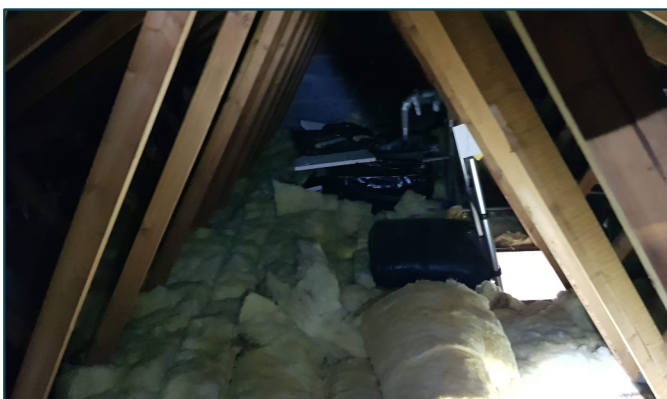
Internal view of loft
