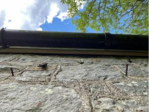
Figure 24: B2 - gaps under timber fascia.
