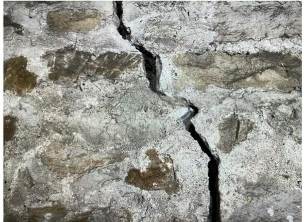
Figure 26: B2 - crack in wall.
