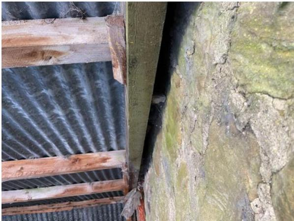
Figure 27: B2 - gaps between timber and wall.
