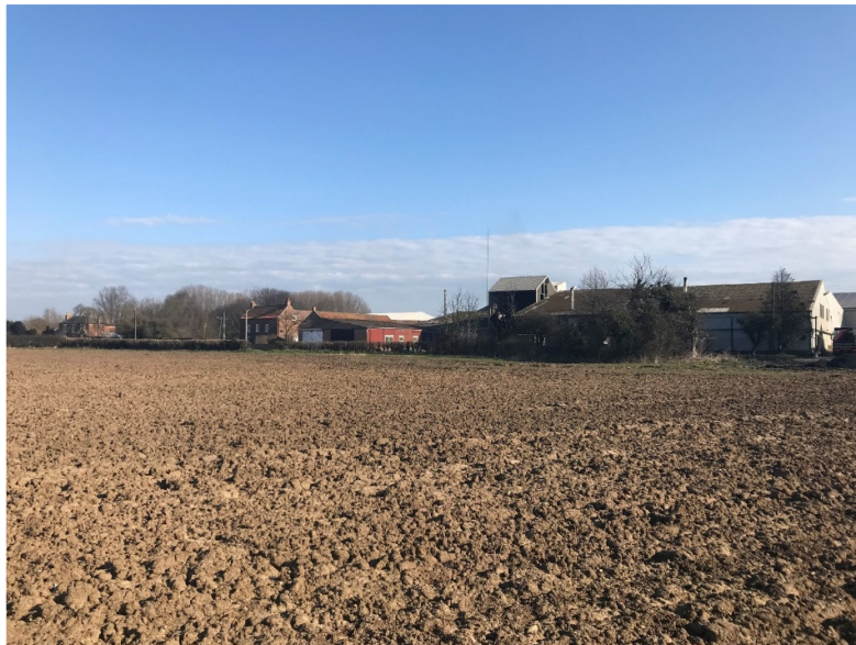
Figure 2: Manor Farm and Manor Farmhouse seen from the application site
