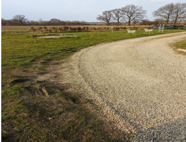
Photograph shows the damage to the grass at the corner of the drive, caused by delivery vehicles using this as a turning point.
