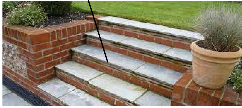
Retaining wall and steps
