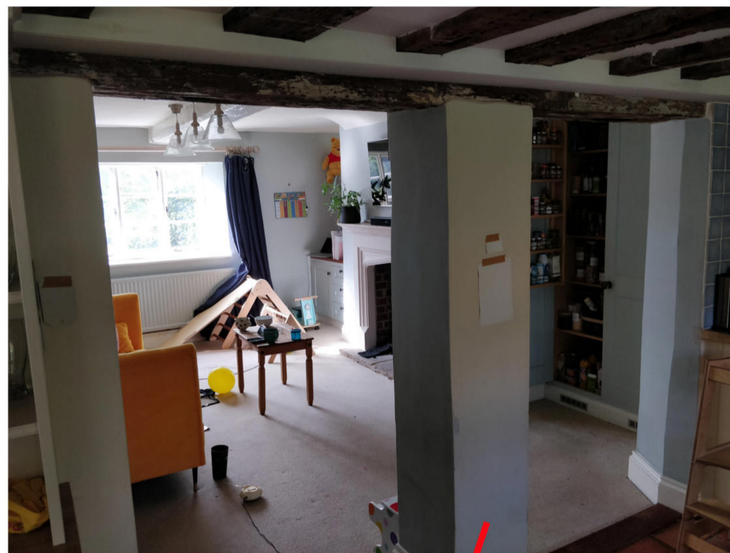
Existing Blockwork Pier
