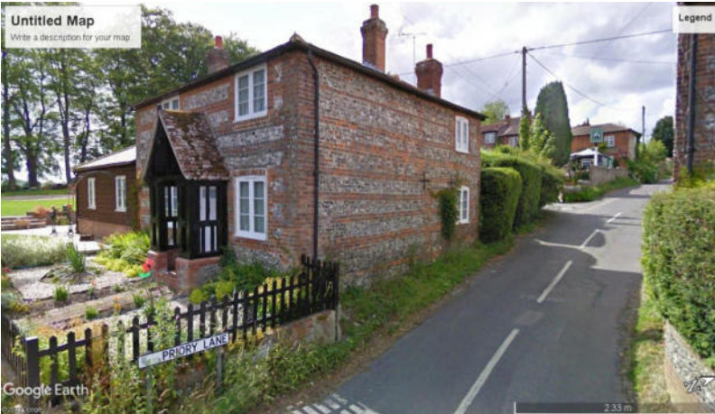
Fig 21029 12A Google View of No.11 Listed Grade2
