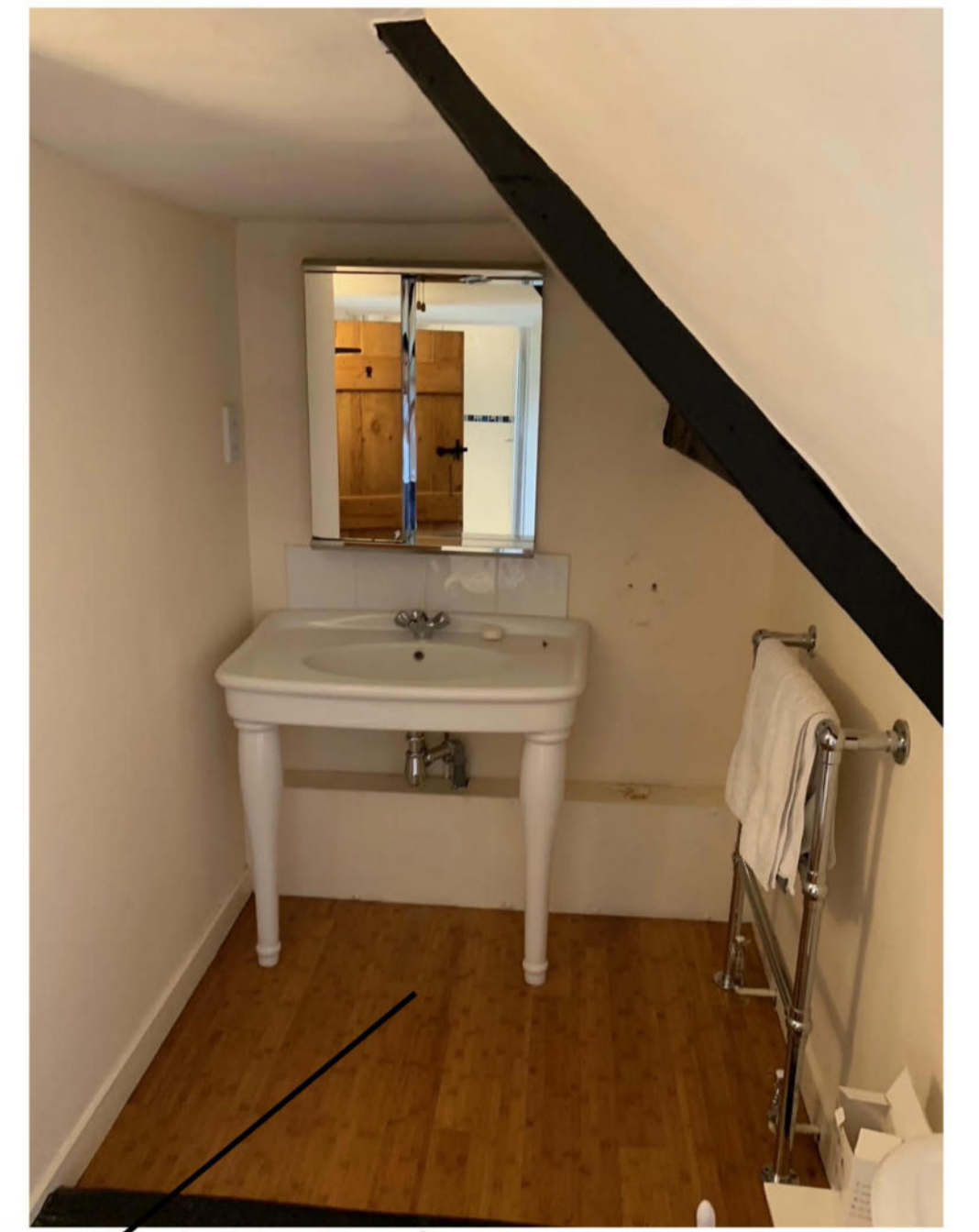
Ex Attic Bathroom
