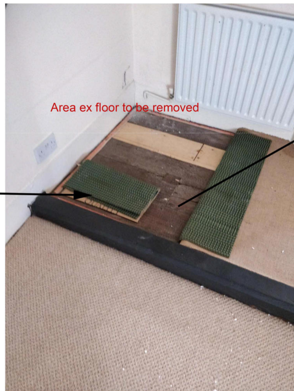
Existing Attic Floor
