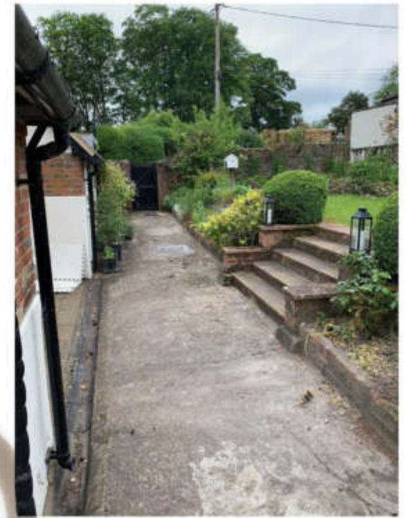
Existing Rear Paved Area
