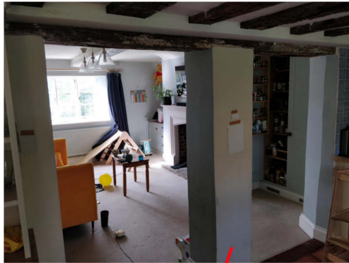
Existing Blockwork Pier
