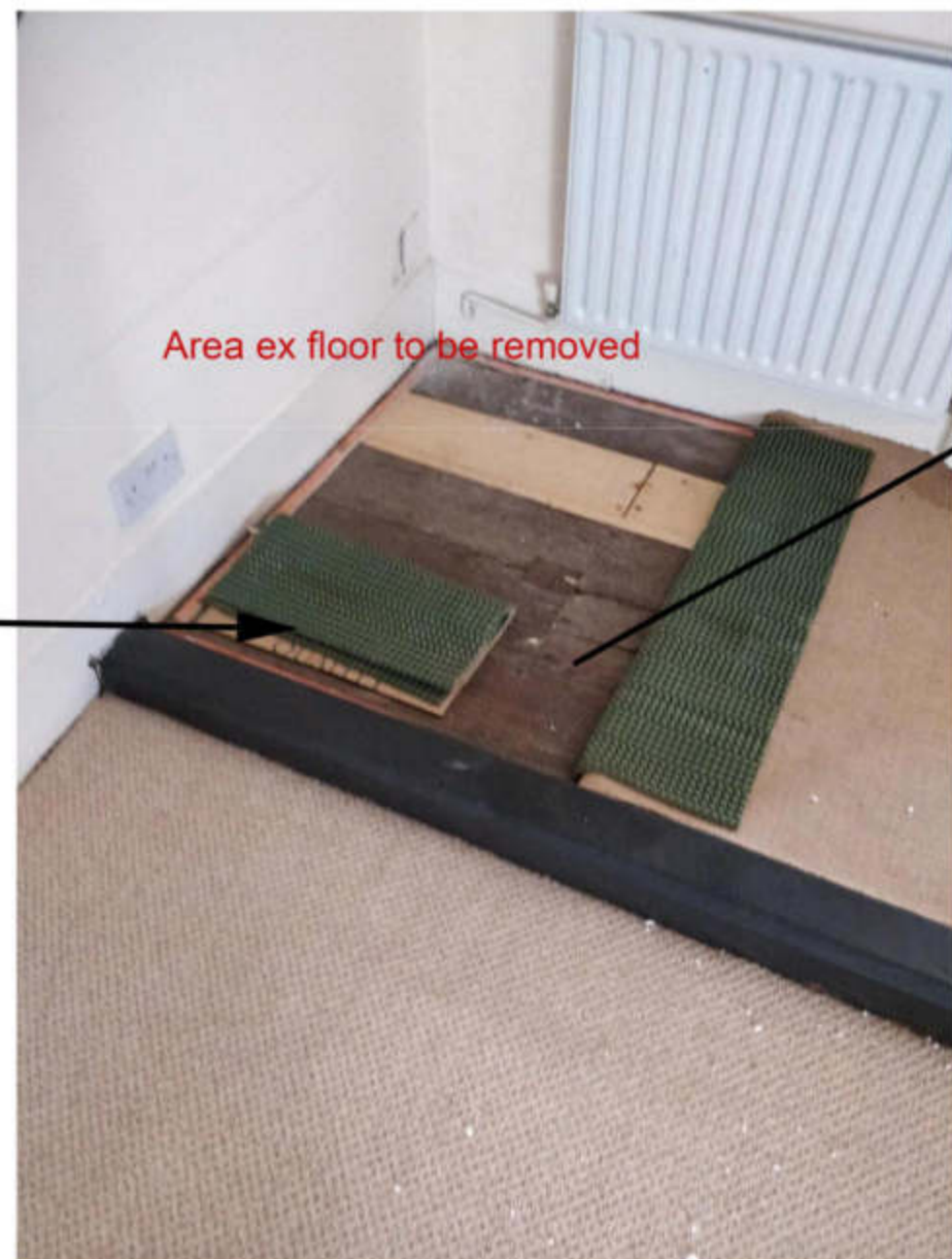
Existing Attic Floor
