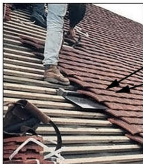
Plain Tile Mech Extract and SVP Ventilation Tile
