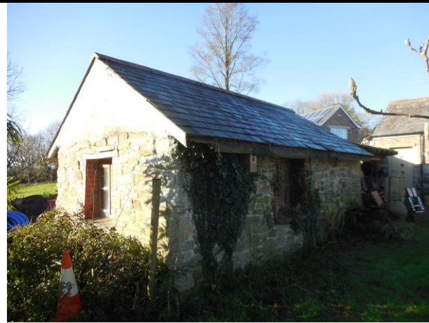
Plate 1. The eastern and southern elevation of the outbuilding
