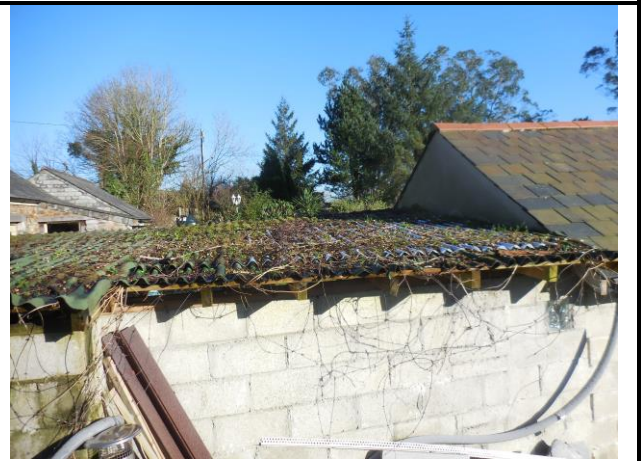
Plate 4. The western elevation of the store
