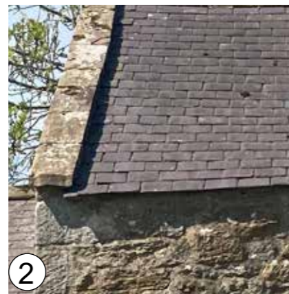
Existing slate roof tiles will be reused where possible
