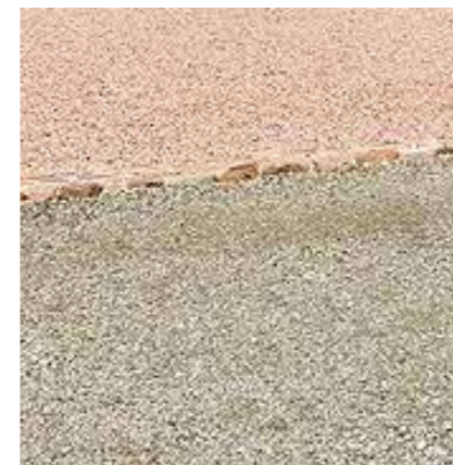
Existing gravel to be reused. Gravel grid grates will be used to ensure longevity.
