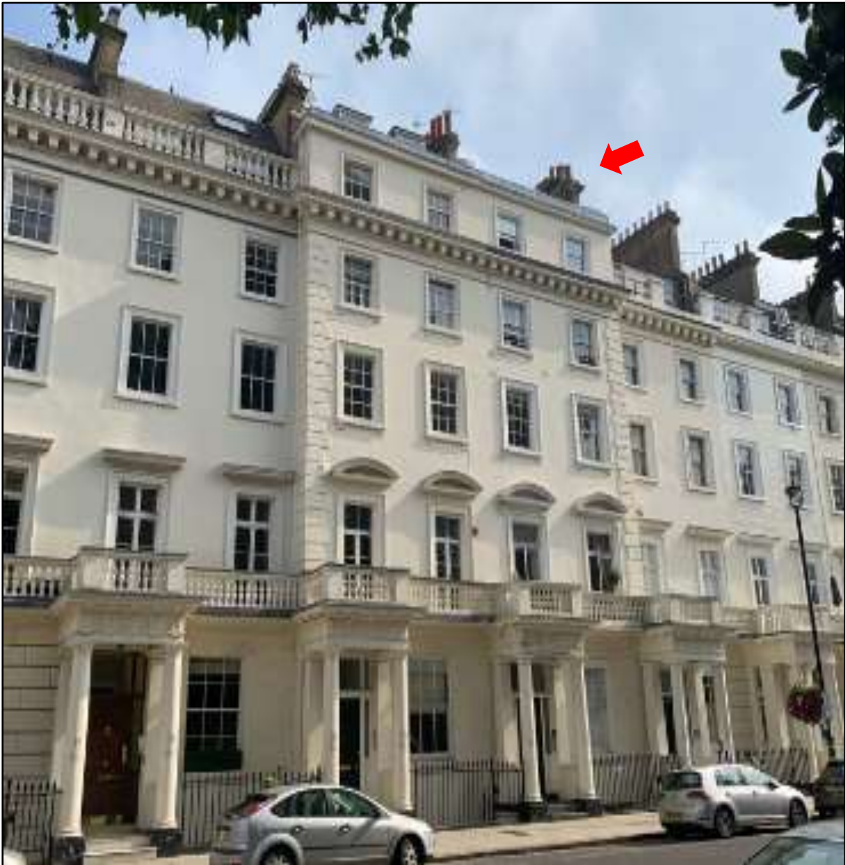
Figure 10: View of the front elevation No. 73 (identified in red).
