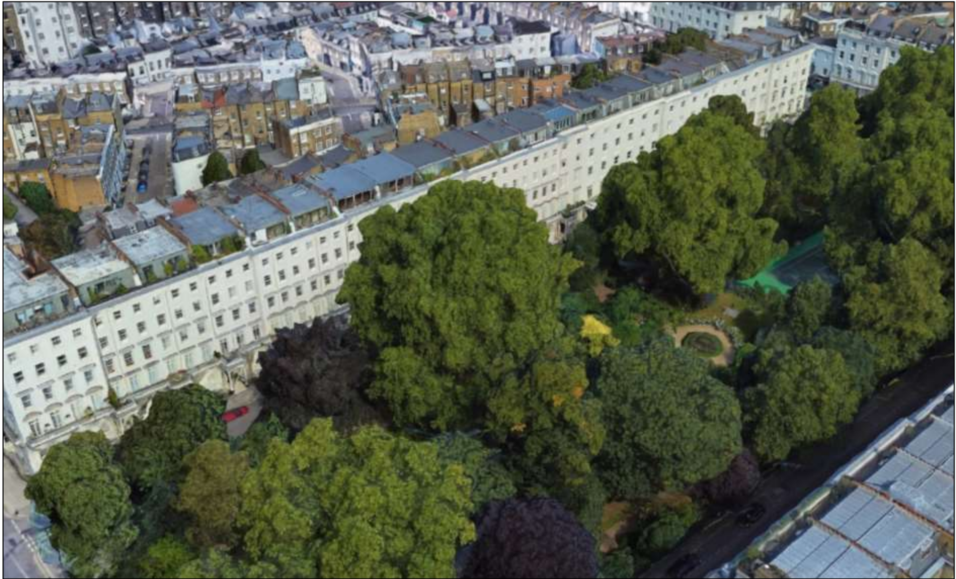
Figure 30: Western terrace of Warwick Square- note the buildings all have roof extensions with varying fenestrations- some with full height glazed windows
