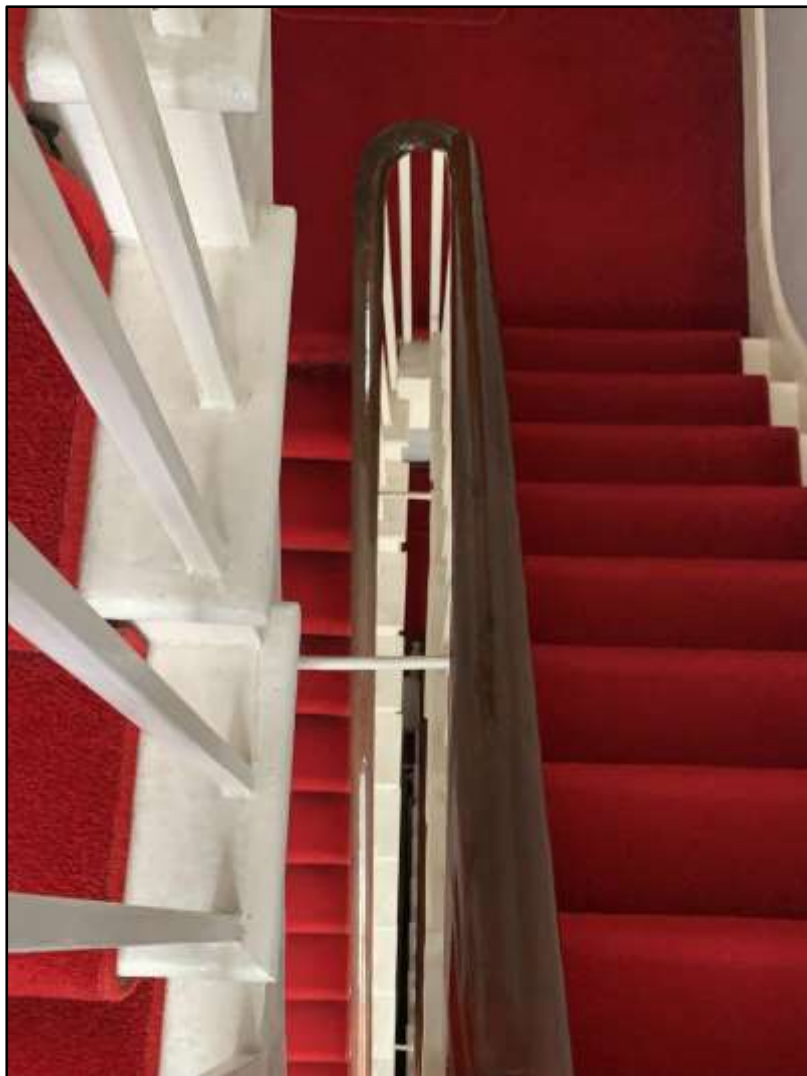
Figure 11: View looking down the original stair that runs throughout the building
