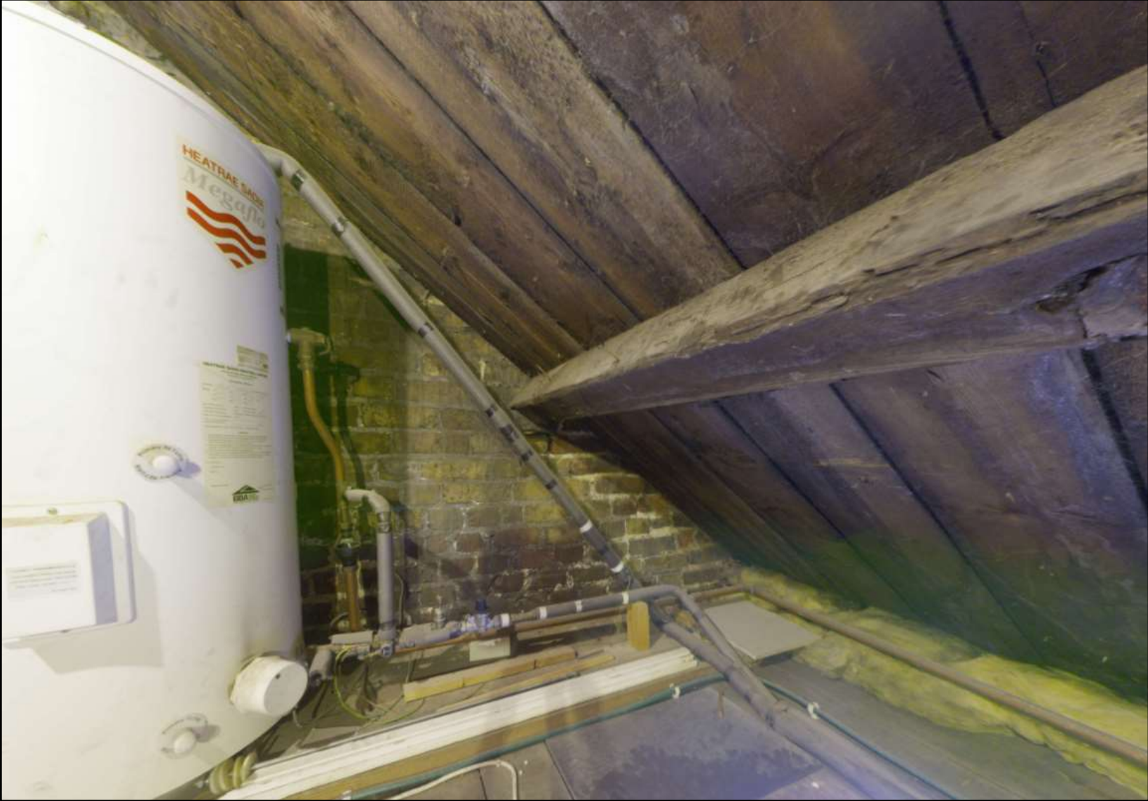
Figure 19: View from inside the attic space
