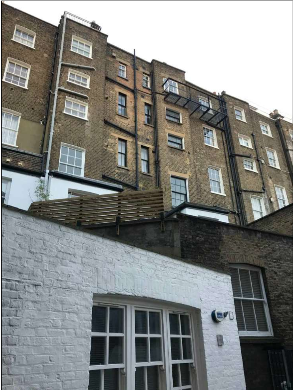
Figure 33: View of the rear of 73 Warwick Square (and the rest of the terrace) from Denbigh Mews- note none of the roofscape is visible
