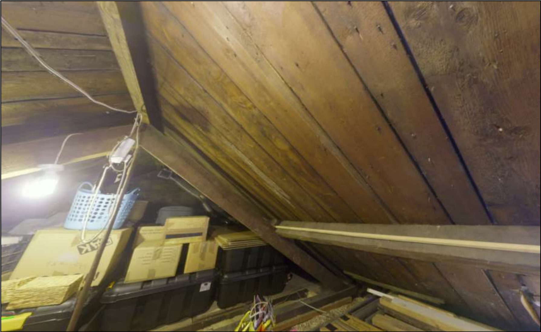
Figure 18: View from inside the attic space
