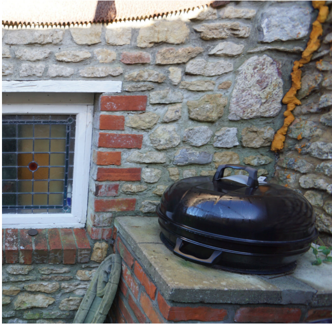
Fig. 5 Existing outbuilding pulling away from the neighbouring wall (built without proper ties) resulting in cracks and leaks throughout the structure. Expanding builders foam used to RHS by previous owner in an attempt to achieve waterproofing.
