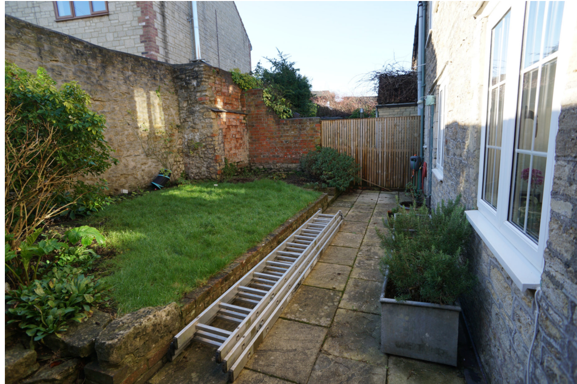
Fig. 2. View of the rear of the house with the patio area to be increased slightly..
