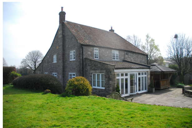
Fig. 4 North west view
