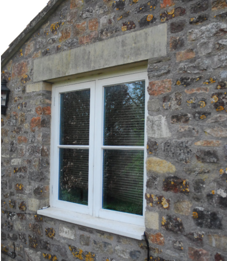
Fig.7 Double glazed casement windows fitted to the 2007 extensions.
