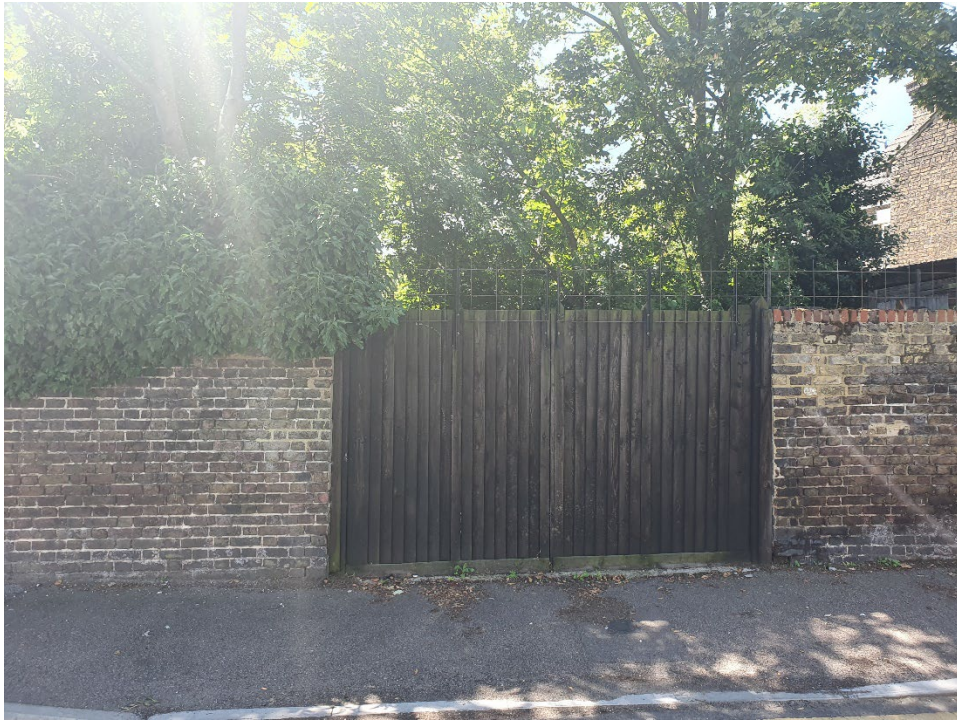
Rear Existing Entrance To Fig Tree House Garden
