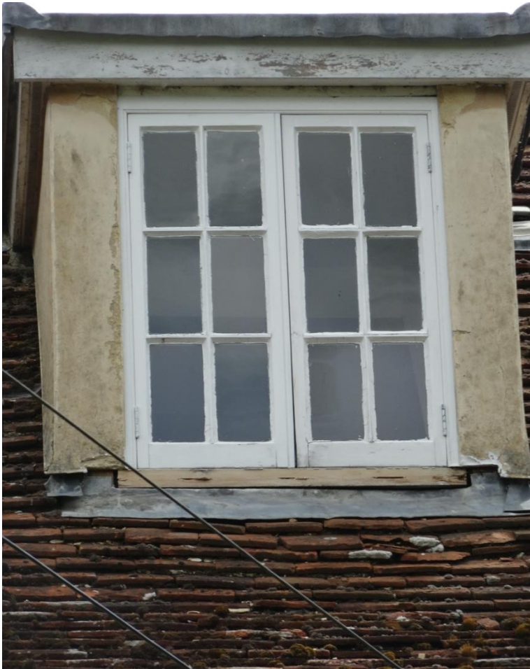
Right dormer window. The sill has already rotted and fallen off.
