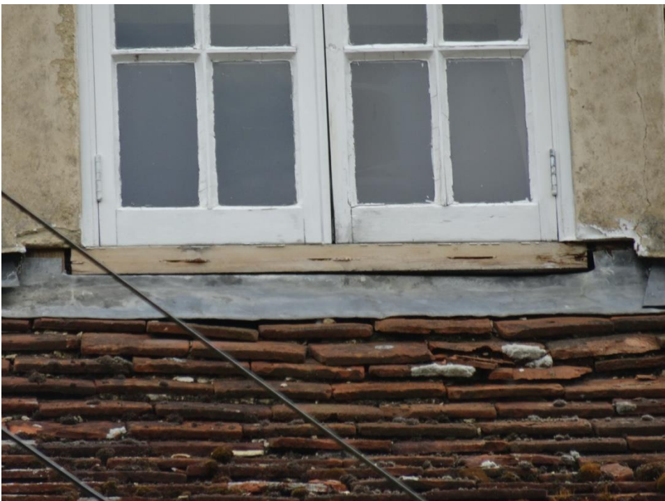
Right dormer window. The sill has already rotted and fallen off.
