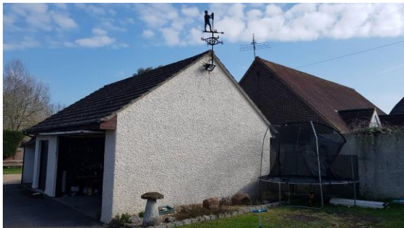
Existing garage and Reubens Meadow adjacent
