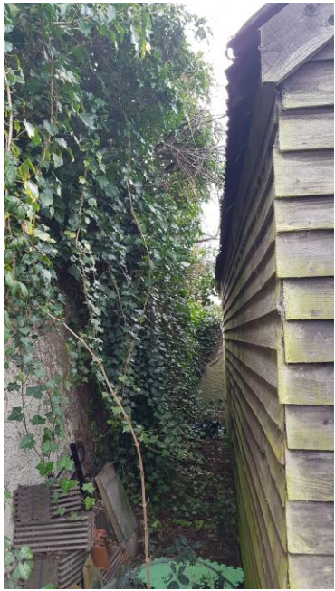
Side boundary wall
