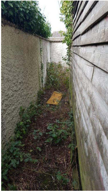
Front boundary wall adjacent shed...
