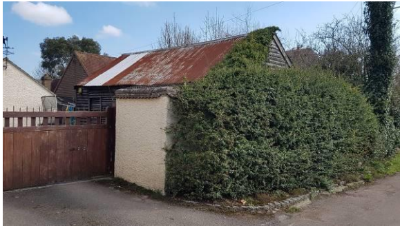
Existing timber shed behind front boundary
