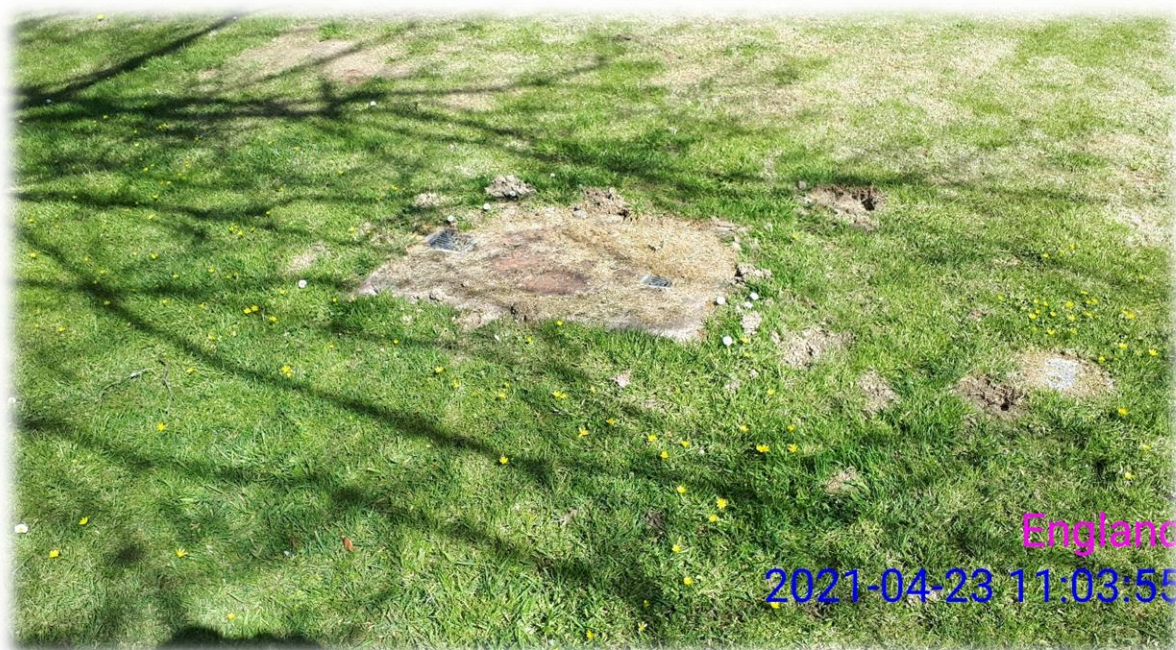
Caravan foul waste disposal and adjacent septic tank
