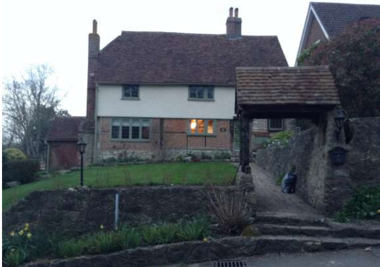
7. Front elevation of Bridge Cottage.
