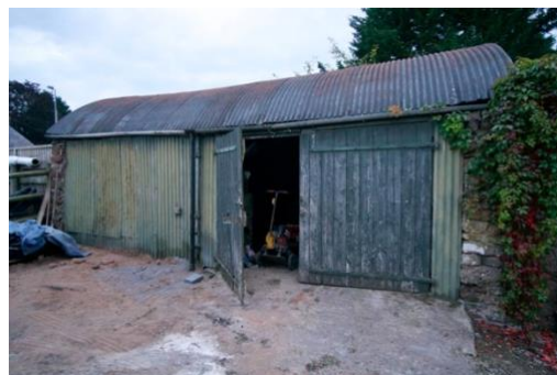
Figure 10 Storage shed N elevation
