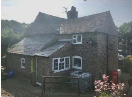
Figure 5 North east gable
