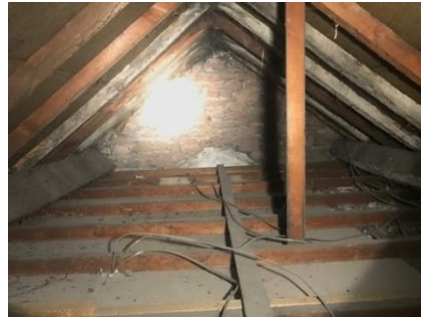
Figure 6 West gable loft space
