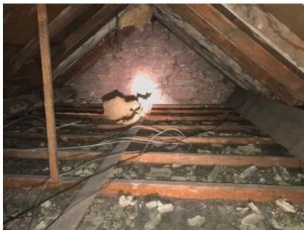
Figure 7 East gable loft space
