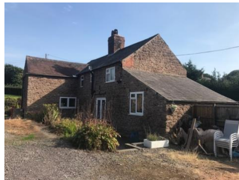
Figure 4 North west gable
