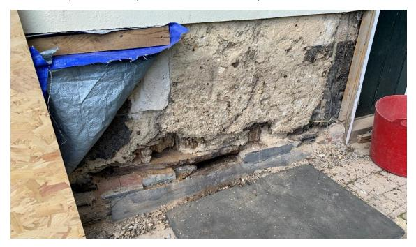
**4.** We propose to fit a new length of plate approximately 2.1m x 125mm x 125mm that will be scarfed adjacent to the crossframe and the studs attached with L-brackets as noted above. The wattle and daub will be repaired with reconstituted clay daub mixed with new wheat straw.
