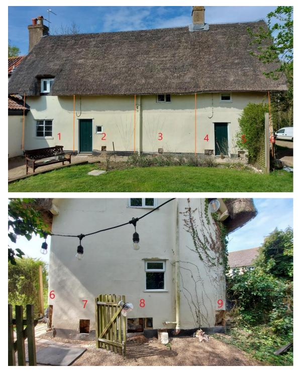
The only section where render was left in place was number 5 – this small section will require the decommissioning of the central heating and hot water boiler and we feel it is crucial for this to remain in service for as long as possible and once work commences, only decommissioned for as short a time as possible. The repair works necessary to this area are very clear and easily understood but will be discussed in order below.
