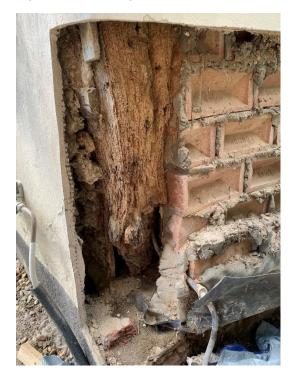
**6.** The southeast corner post (left) will be scarfed with a new section of oak, approx. 700mm long x 160mm x 180mm using a simple half-lapped scarf joint approximately 250-300mm long and fixed with M10 stainless steel coachscrews.
