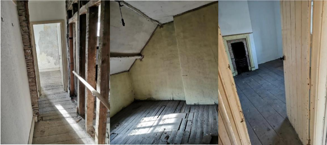
Typical Interiors to Cottage nos. 1 and 2
