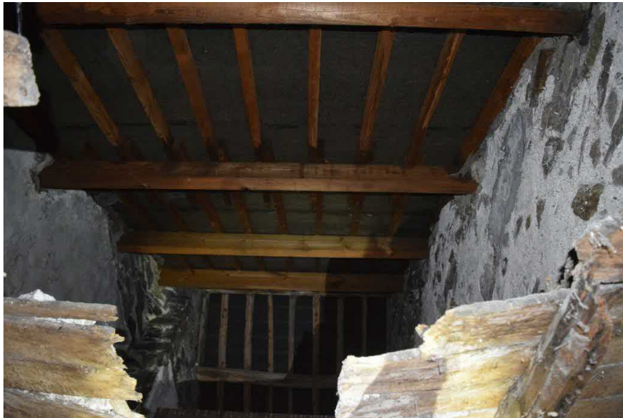
Figure 4.8. View of roof over cottage three
