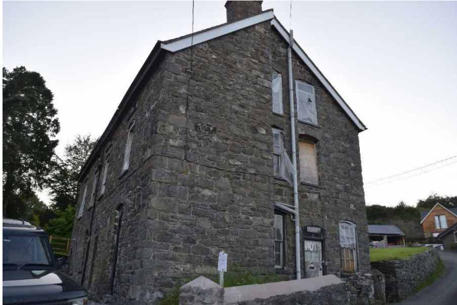
Figure 4.3. Building from the east
