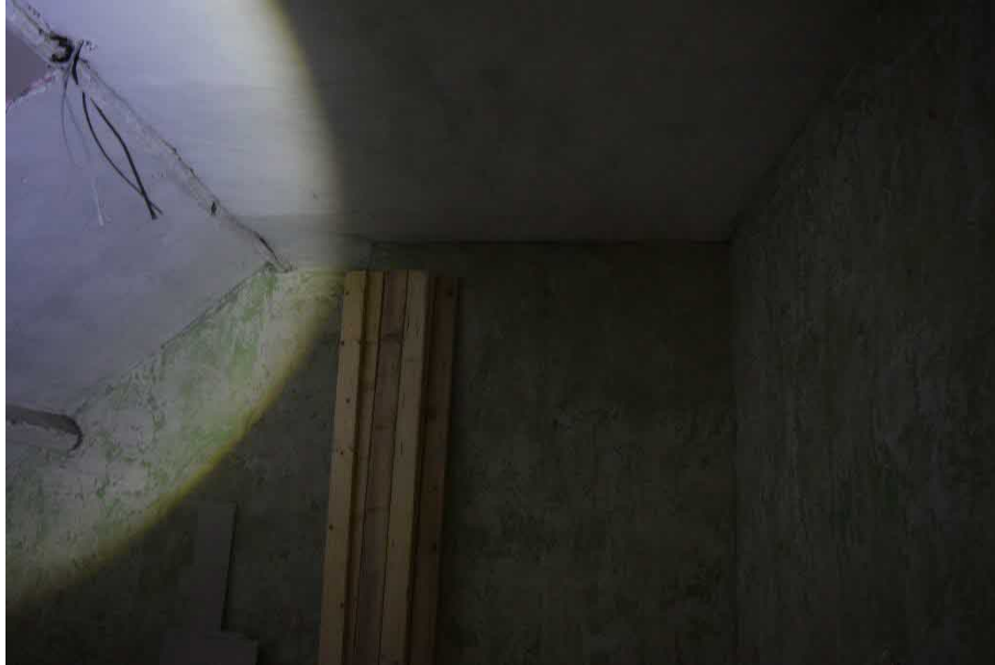
Figure 4.6. Showing ceiling on second floor
