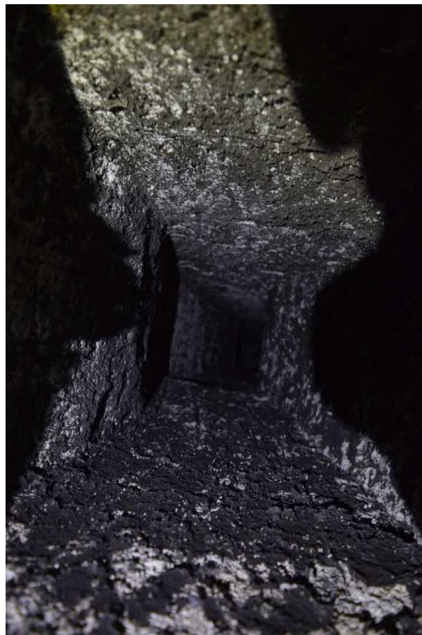
Figure 4.7. View up chimney
