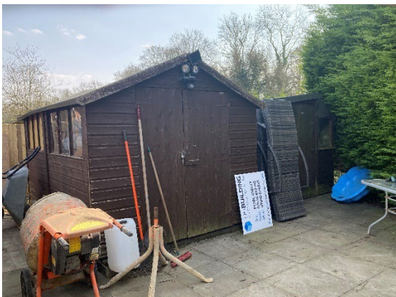
Existing sheds and garage to be demolished
