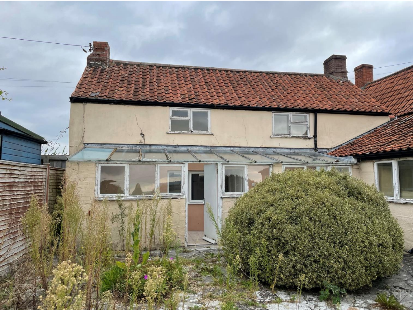
Figure 2 View to rear
