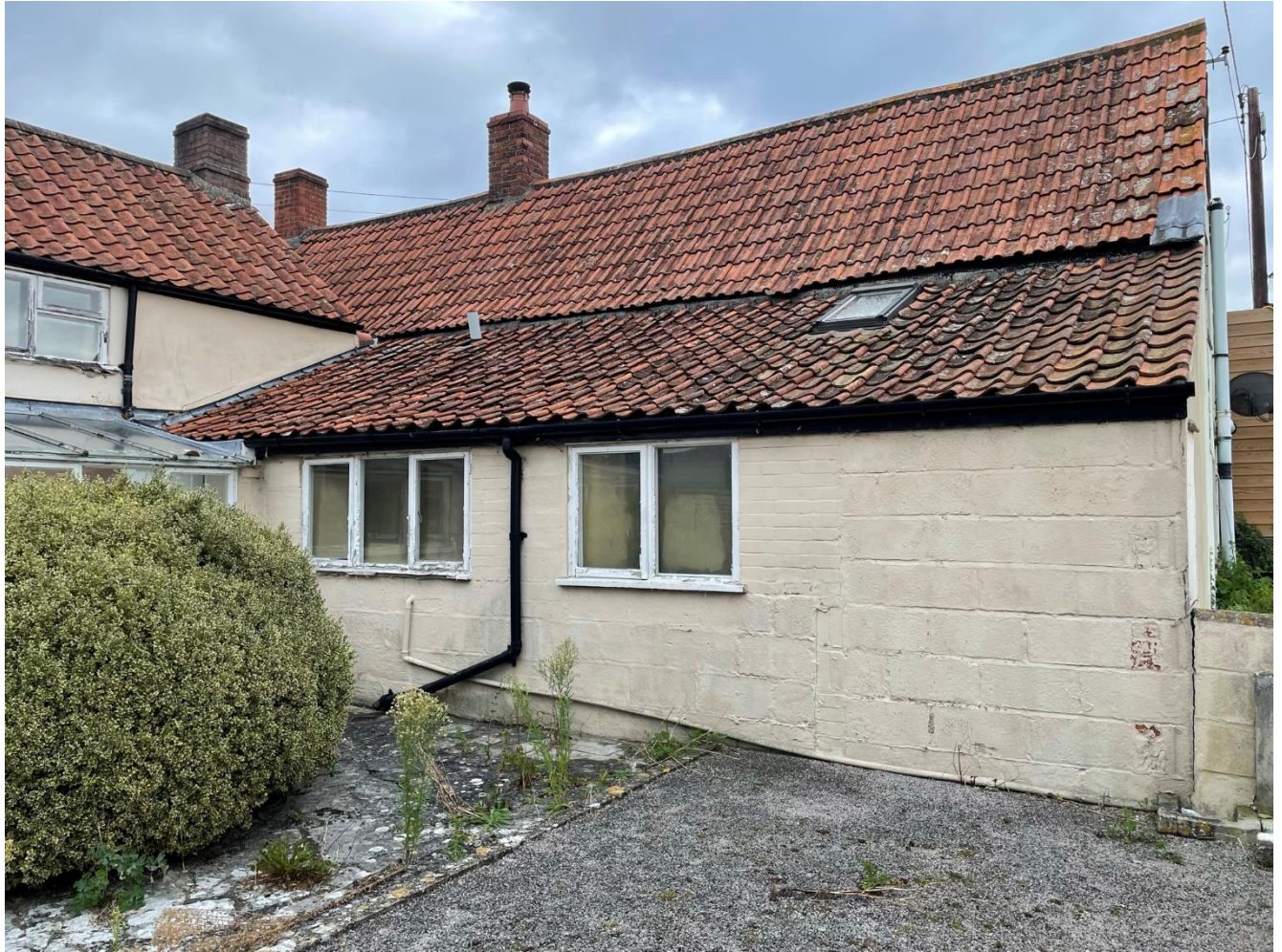
Figure 3 Existing Rear Extension
