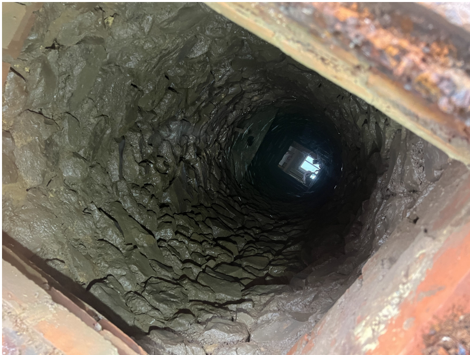
Fig 6 Well in room 6 showing brick encasing iron frame and cover.
