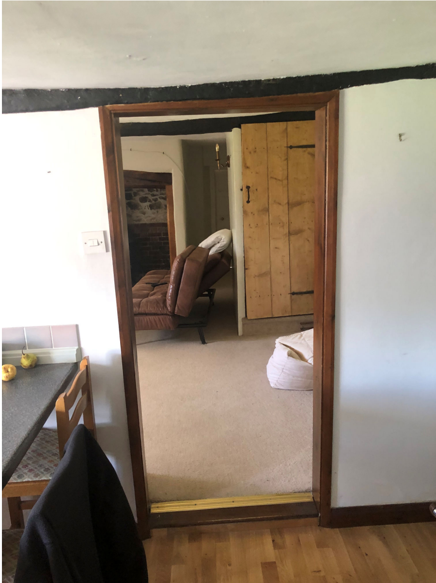
Fig 3 view from room 2 into room 3 showing replacement door to stair in original frame.
