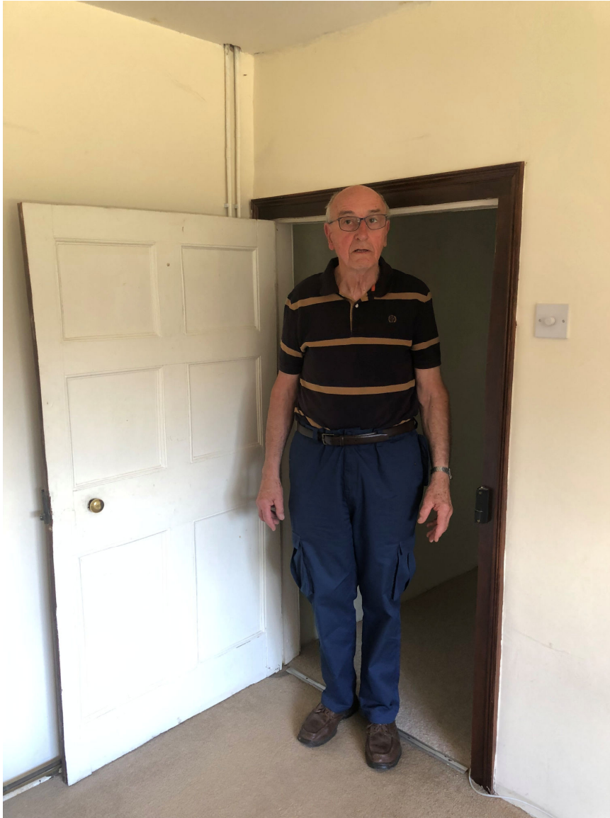
Fig 10 showing low door from room 10 to head of stairs. Door frame to be raised and bottom of existing door and frame extended 150mm.
