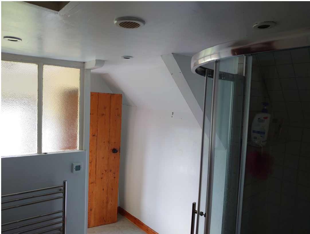
Fig 7 Showing 20 th C glazed partition and shower etc. to be removed.
