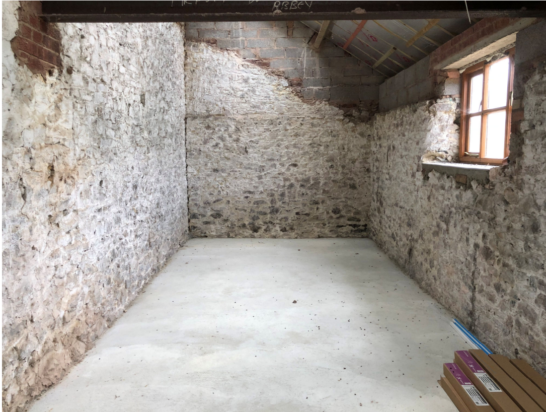
Fig 5 showing wall on left to have new opening in to room 4
