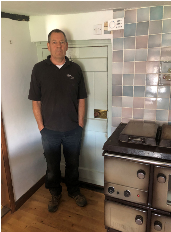
Fig 1 Door from room 2 to room 6 showing restricted height and Rayburn in front of original fireplace.
