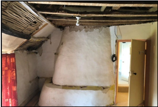
First floor fire place: image 4.0
