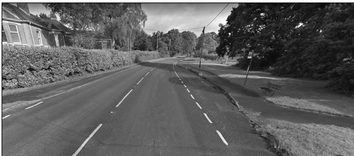
Figure 3.2 – A36 Footway and Crossing Point
