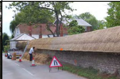
Thatched cob walling restoration at Longparish
