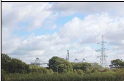
Waterside cranes and high voltage power lines loom over wooded horizons – nr. Marchwood
