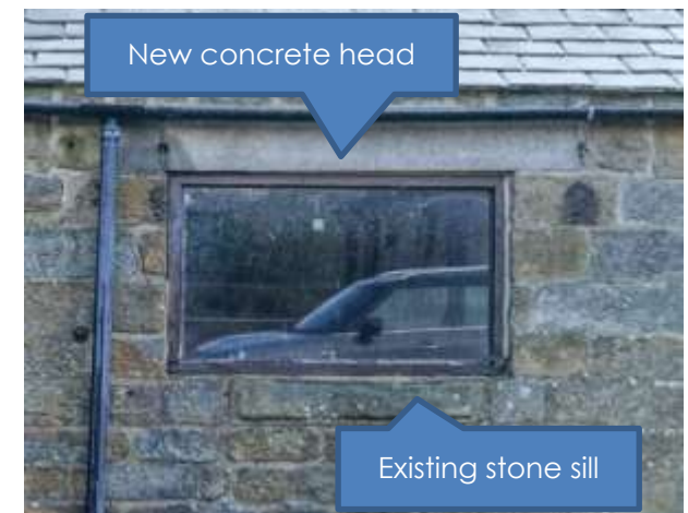
Fig. 12. Window on Western facade
