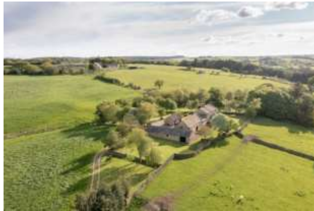
Fig. 6. Aerial view from the East
