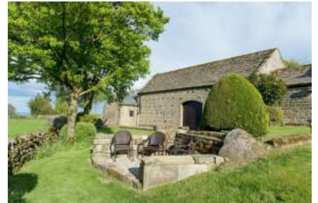
Fig. 7. Barn - North elevation
