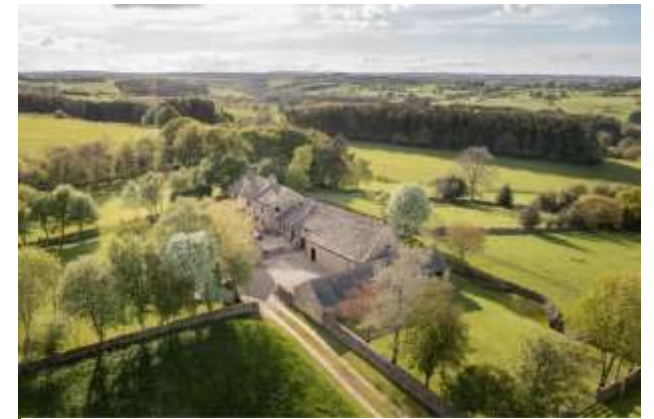
Fig. 10. Aerial view from the East
