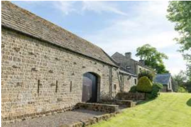
Fig. 5. Barn - North elevation
