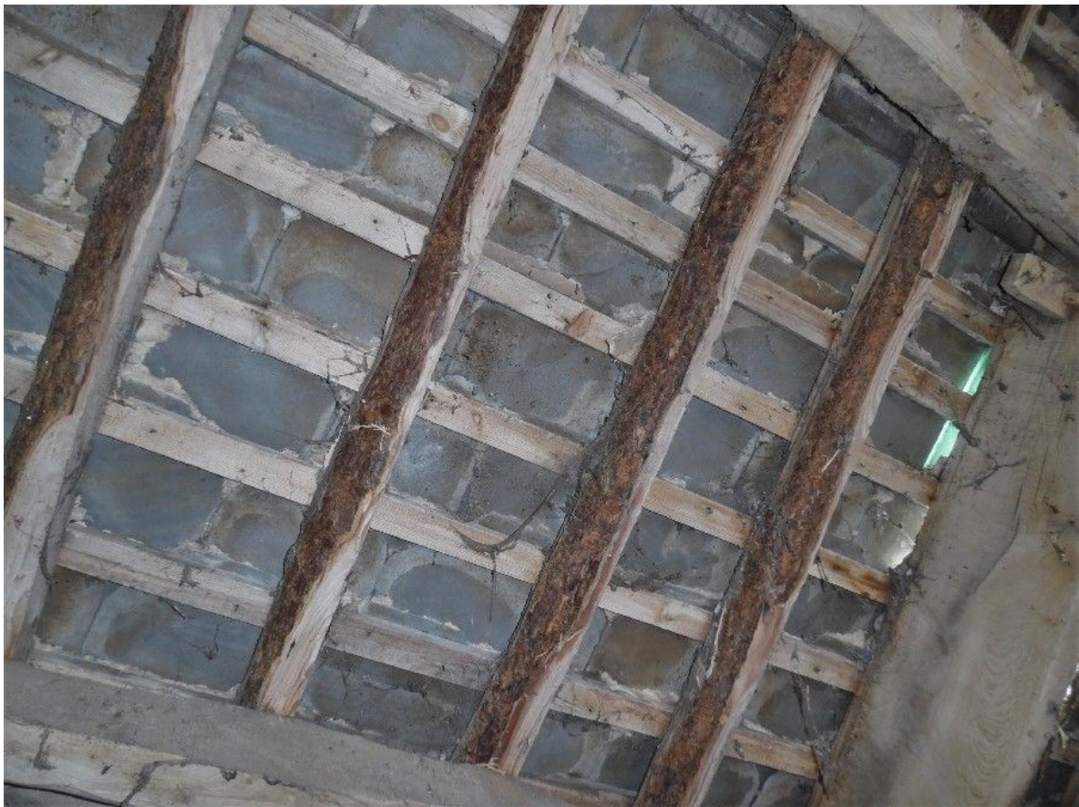
Plate 6: Typical roof rafters. Possibly tree branches or small trunks.
