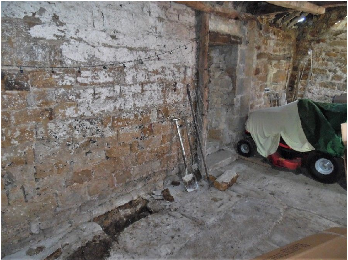
Plate 9: Slab within the barn.
