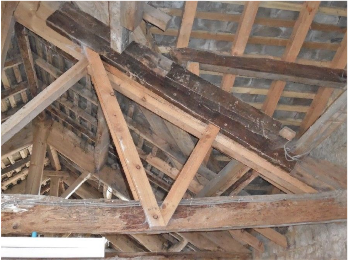
Plate 7: Strengthening of original timber king post truss.
