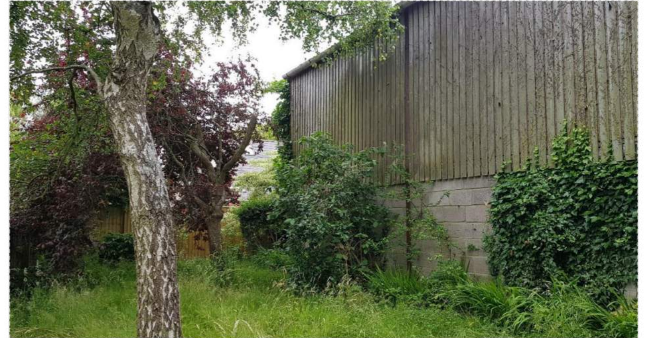
Northwest elevation - Timber cladding above concrete blockwork
