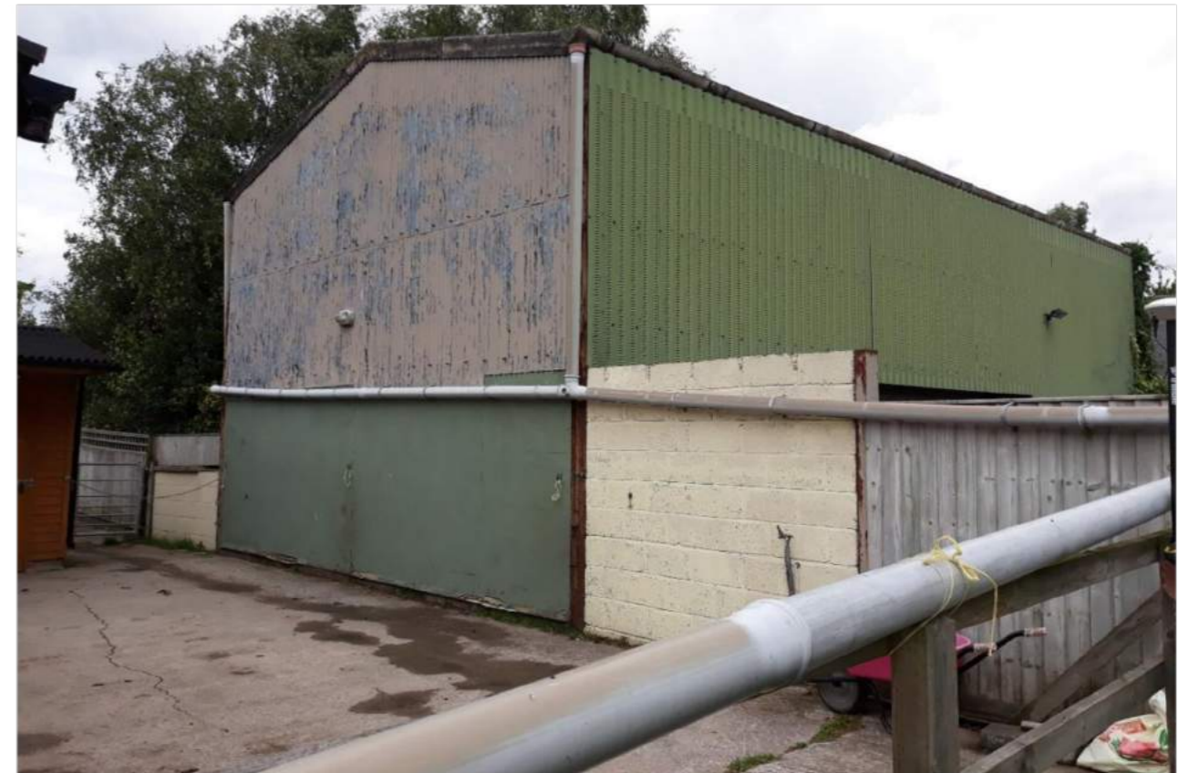
Southwest elevation - Corrugated metal cladding above concrete blockwork
