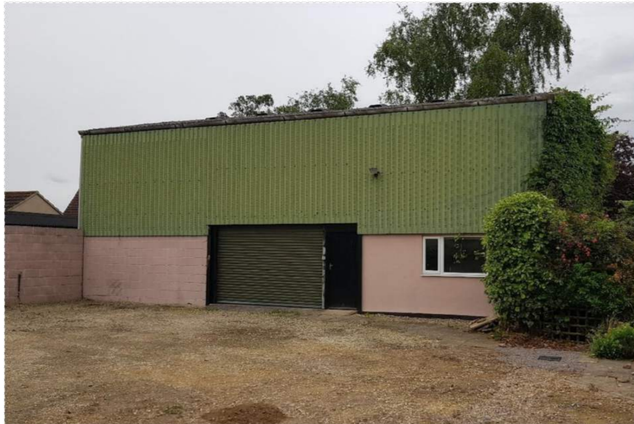
Southeast elevation - Louvered cladding above concrete blockwork
